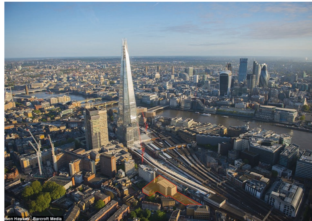
Figure 2.2 Aerial image Site Location, London Bridge
