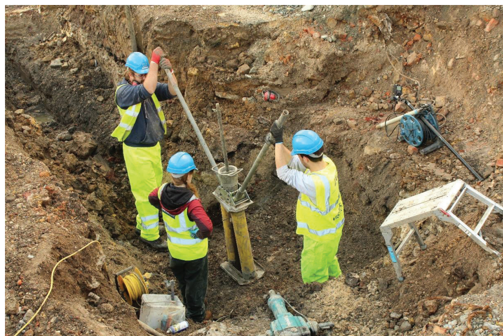
Plate 2: Excavation of Borehole 4 in Trench 2, looking west.
