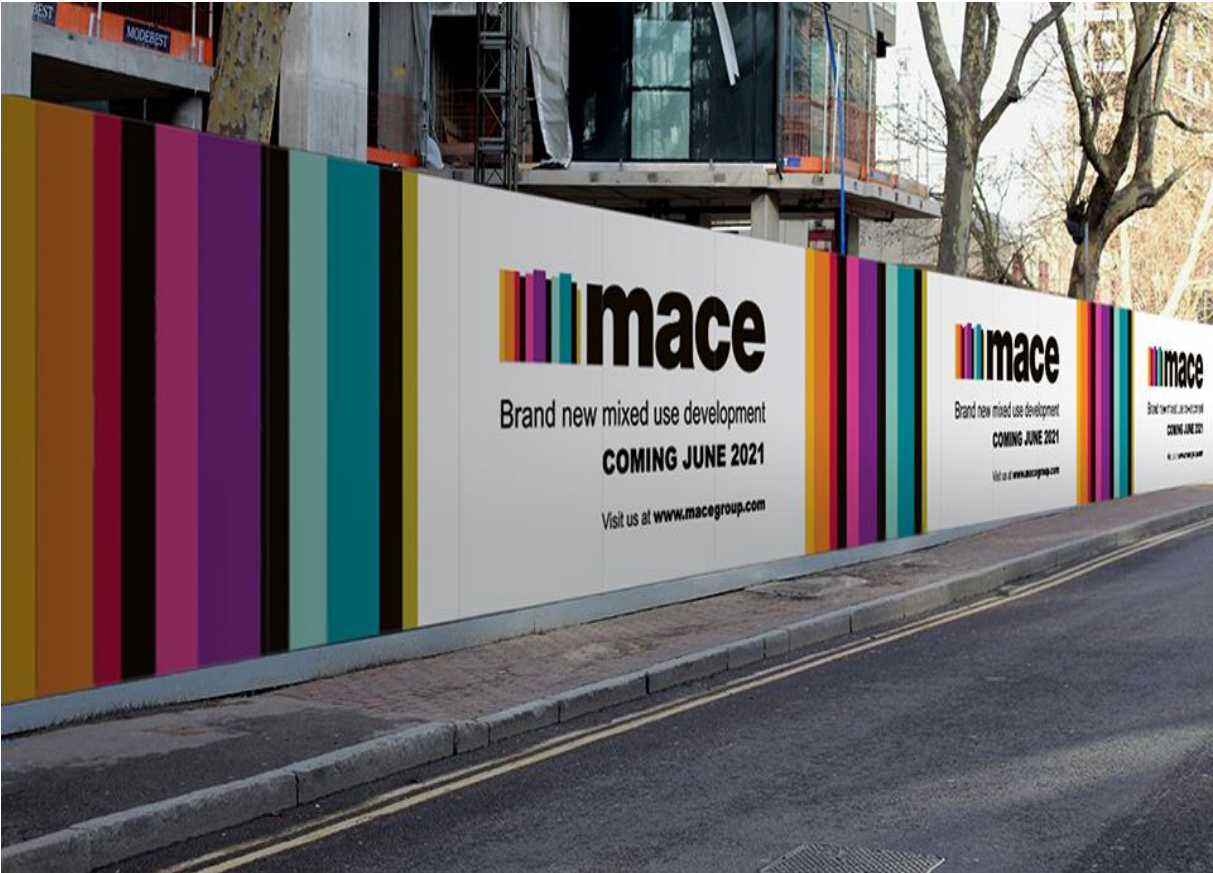
Example of construction security hoarding
