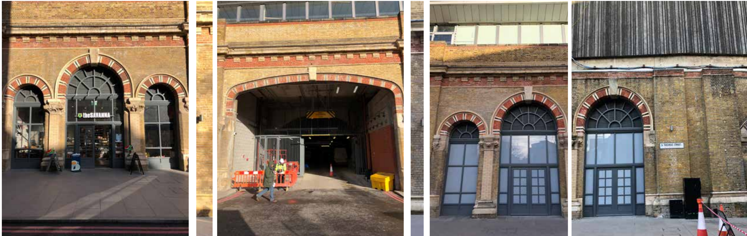
London Bridge Station. St Thomas Street view looking north
