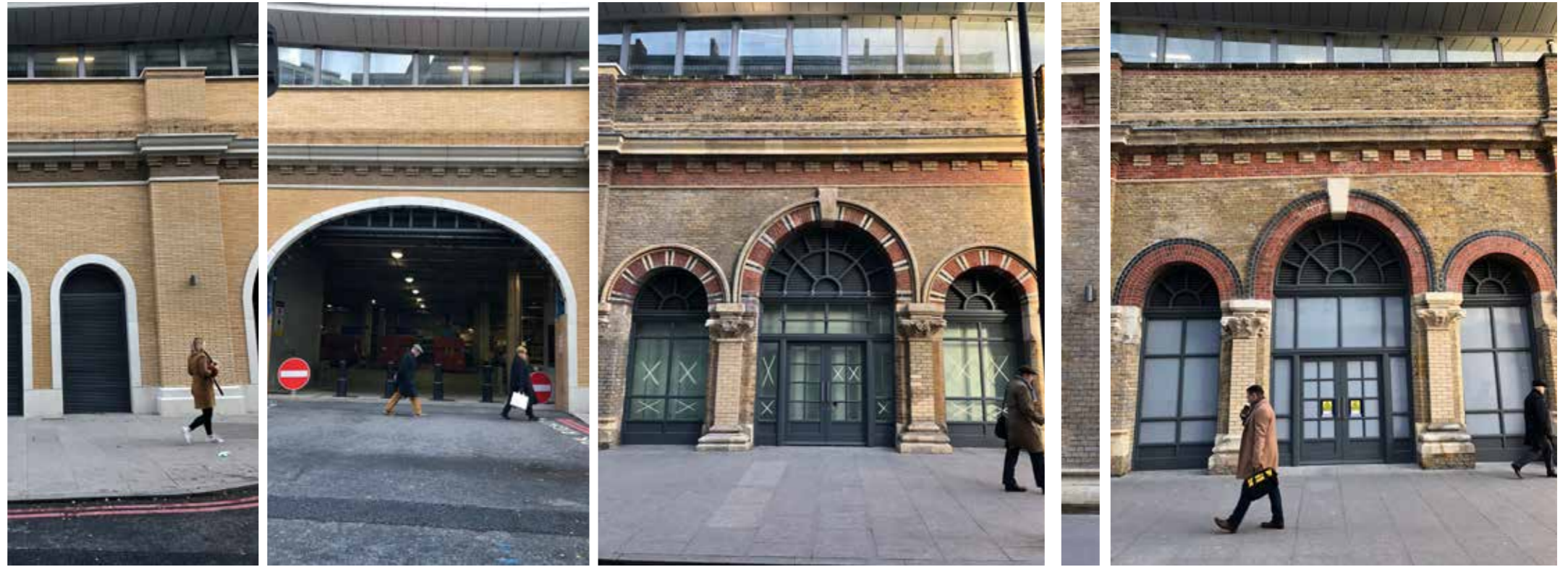
London Bridge Station. St Thomas Street view looking north
