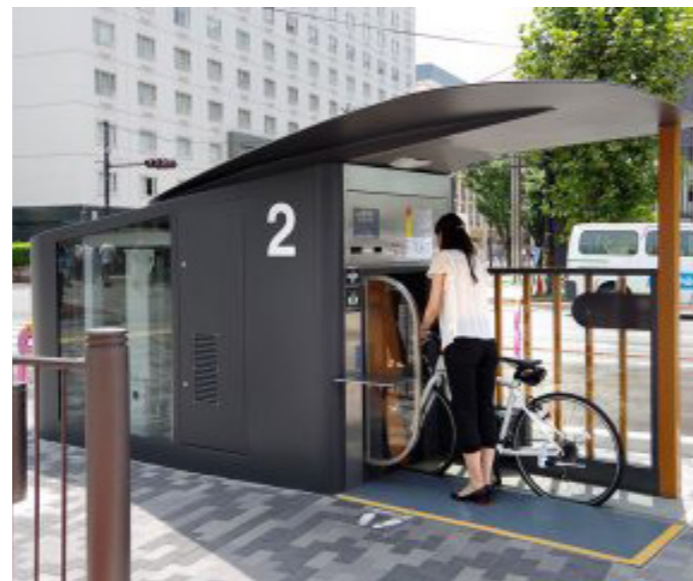
Case Study installation of below ground cycle store interface in Japan
