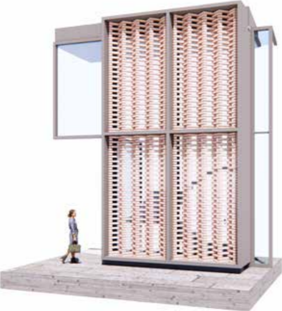
Infill Building Brick Screen Facade
