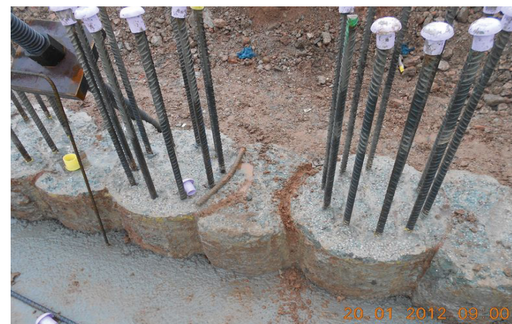
Figure 7.3 Site construction example of secant wall
