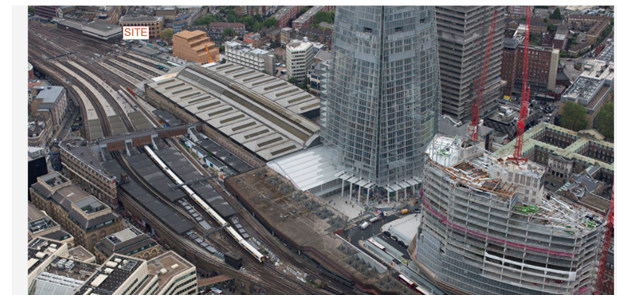
Figure 3.8 Aerial view of site and Network Rail compound
