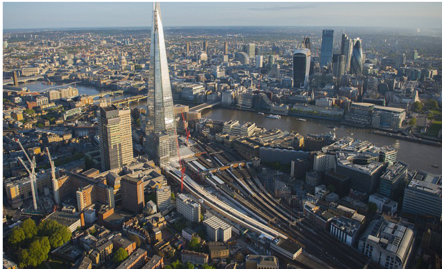
Figure 3.1 Aerial view looking north capturing The Shard, Guy's and St Thomas' Hospital and London Bridge Railway Station.
