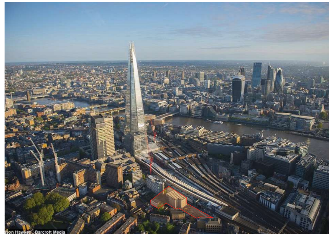
Figure 2.2 Aerial image Site Location, London Bridge
