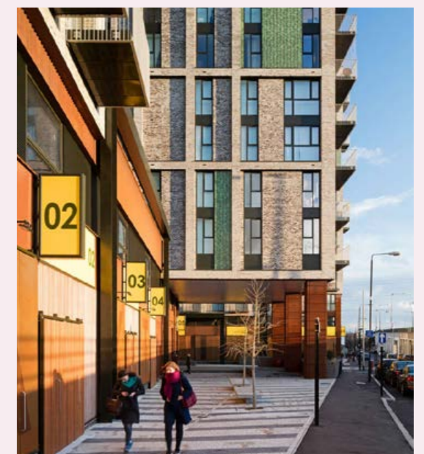
FIG 4.28 Caxton Works combines light industrial units at ground floor level with residential above demonstrating the potential for forward thinking and bold mixed-use typologies in the capital. Image credit: Studio Egret West
