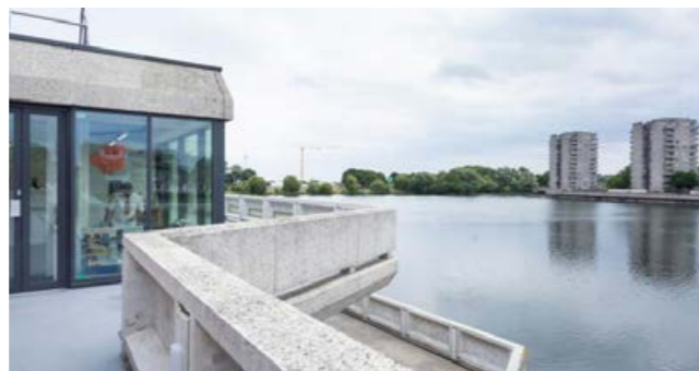
FIG 3.24 Lakeside Centre was reopened by Bow Arts, and funded by the Mayor of London and Peabody. It includes new affordable creative workspaces, a cafe, early years day nursery run by the YMCA, and space supporting SMEs and start ups. Photo credit: Bow Arts.
