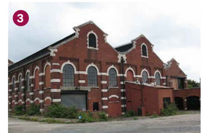
FIG 4.24 Plumstead Power Station - RB Greenwich and the Mayor of London are funding a project to bring the Grade II Listed building back into use to benefit the area and local economy. Photo credit: Stephen Craven
