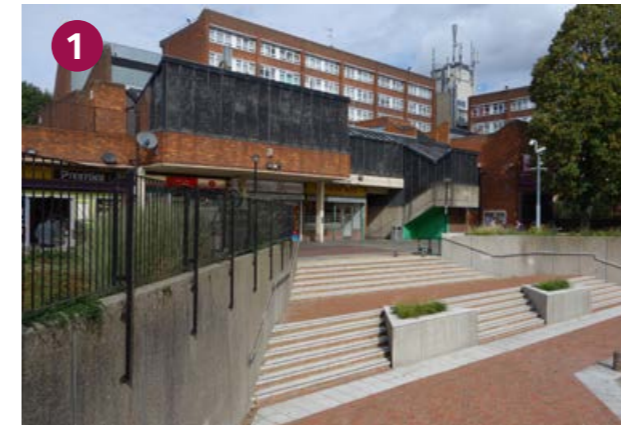
FIG 4.44 The Mayor of London granted £1.15 million through the Good Growth Fund to improve the public realm and buildings in the Moorings to create a community, enterprise and learning hub for Thamesmead
