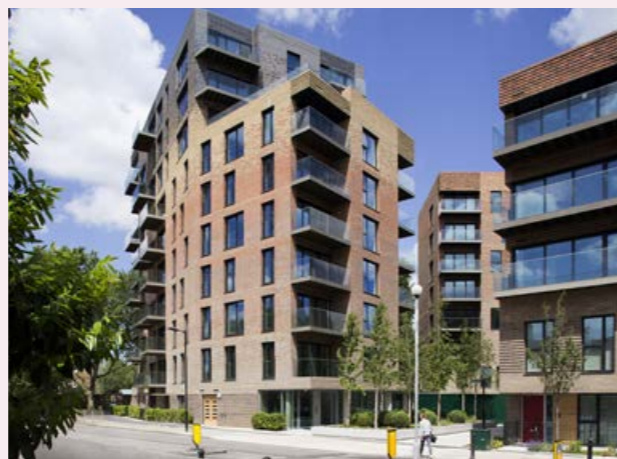
FIG 4.39 High-quality apartments integrated with a new landscape and play spaces. Public space is a key aspect of the project, with accessible landscaping, a pedestrianised link across the site and generous play spaces throughout the development. Photo credit: Alex de Rijke.
