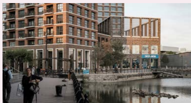
FIG 4.40 Canada Water is transformed from an out-of-town shopping area to a new mixed-use town centre that has the intimacy and animation of a traditional high street. Photo credit: Tim Crocker.
