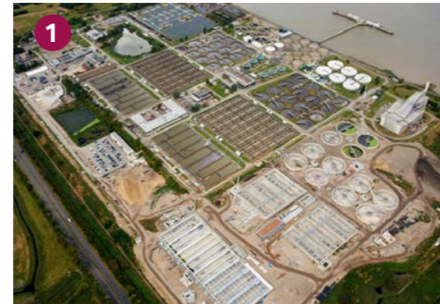
FIG 4.64 Crossness Sewage Treatment Works is the second largest waste treatment plant in Europe
