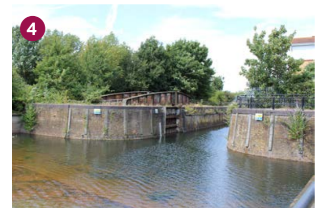
FIG 4.25 The Lock and Swing bridge at Broadwater Dock is Grade II Listed. Although it is a prominent local feature, it is not publicly-accessible.
