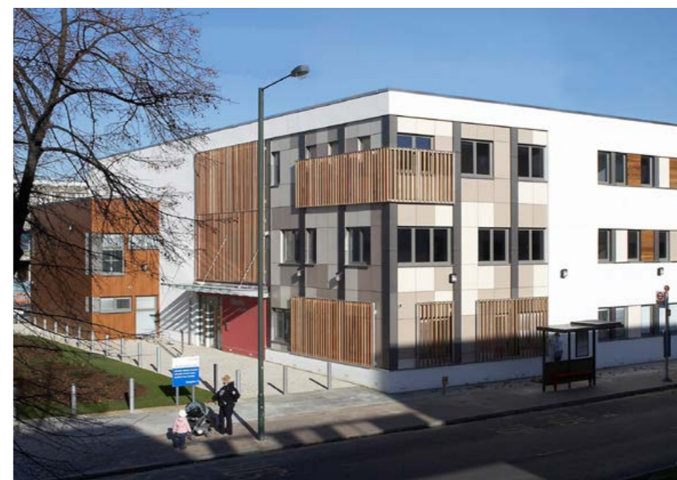
FIG 3.42 Lakeside Medical Practice. Photo credit: sonnemann toon.
