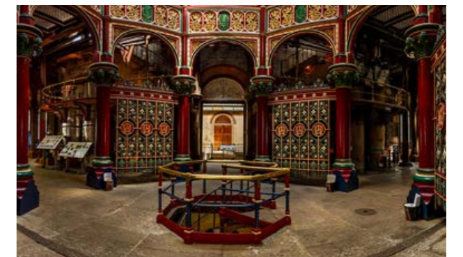
FIG 3.26 Crossness Grade I listed pumping station sits on the Thames Path but suffers from poor accessibility - this is beyond the OA but is recognised as a local asset
