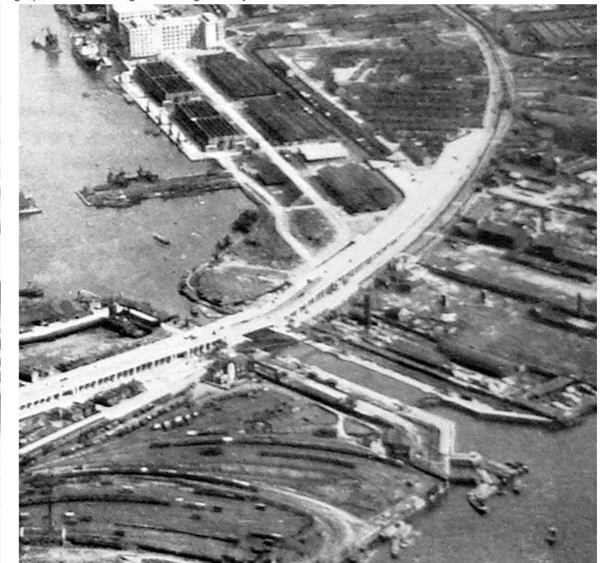
Aerial photograph (c.1935) showing the ship canal and railway lines
