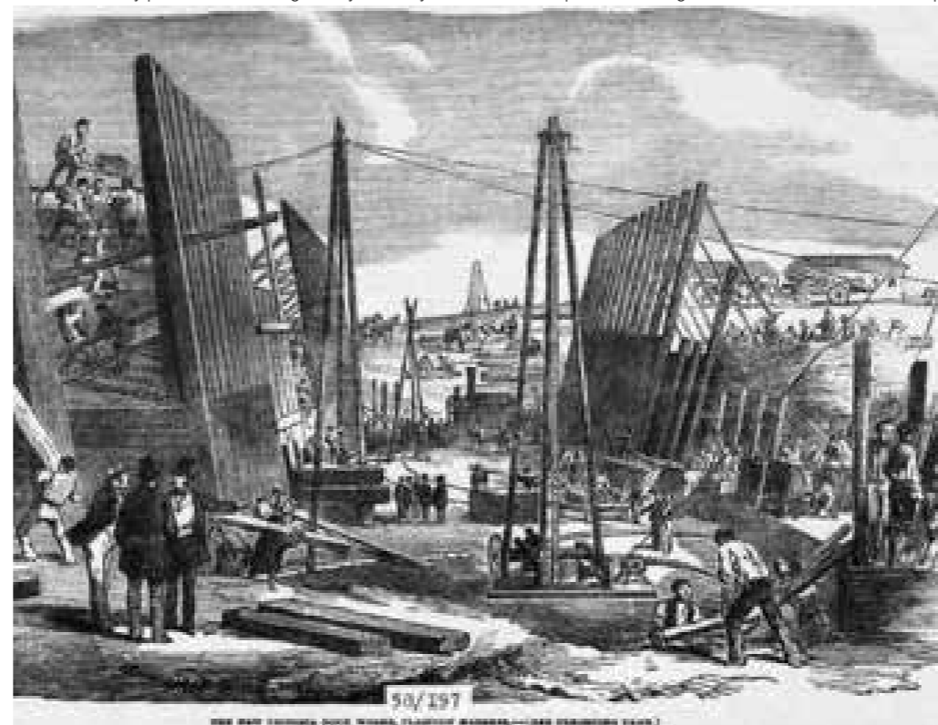
Illustration (1854) showing workmen building the Victoria Docks
