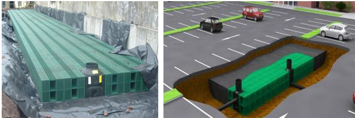
Figure 4: Typical Cellular Attenuation Tank
