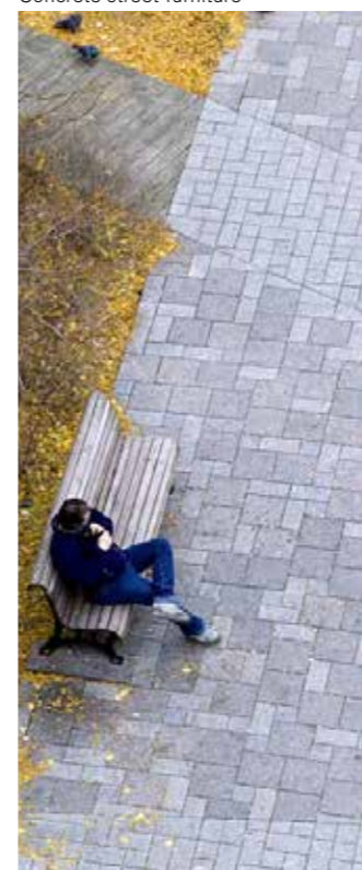
Blocks of different size paving
