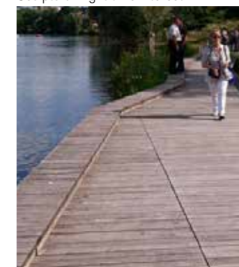
Timber boardwalk jetties
