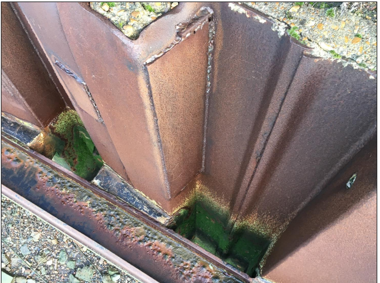
Figure 3.1: Typical photograph of upper level of river wall, showing steel plate repairs to sheet piling, taken from the land side of the river wall
