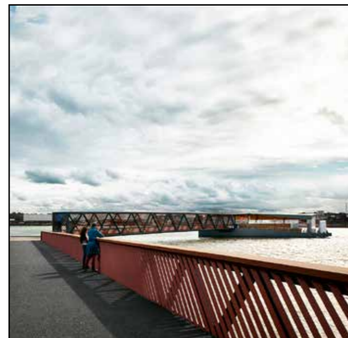
New River bus jetty at Royal Wharf Pier
