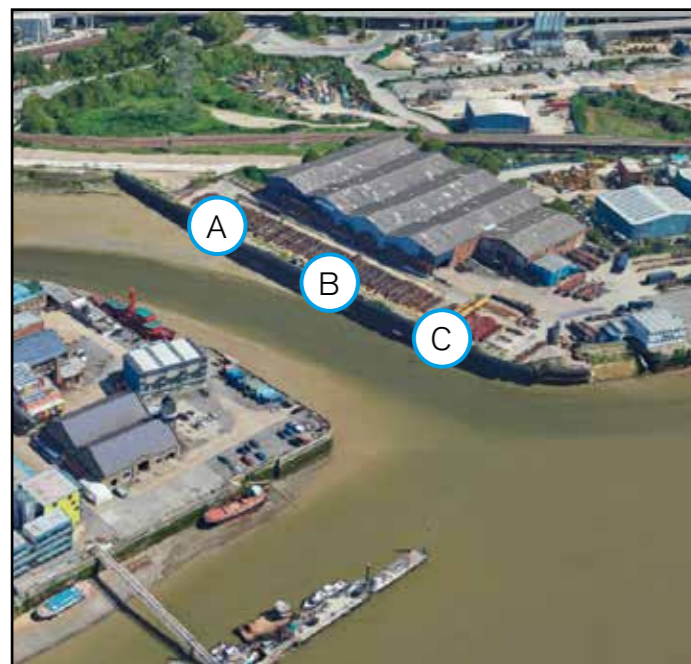
Existing River Lea showing potential bridge landing points
