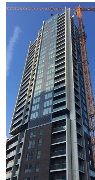
Stratford Edge Bolt-on balconies with non-structural side panels to level 29
