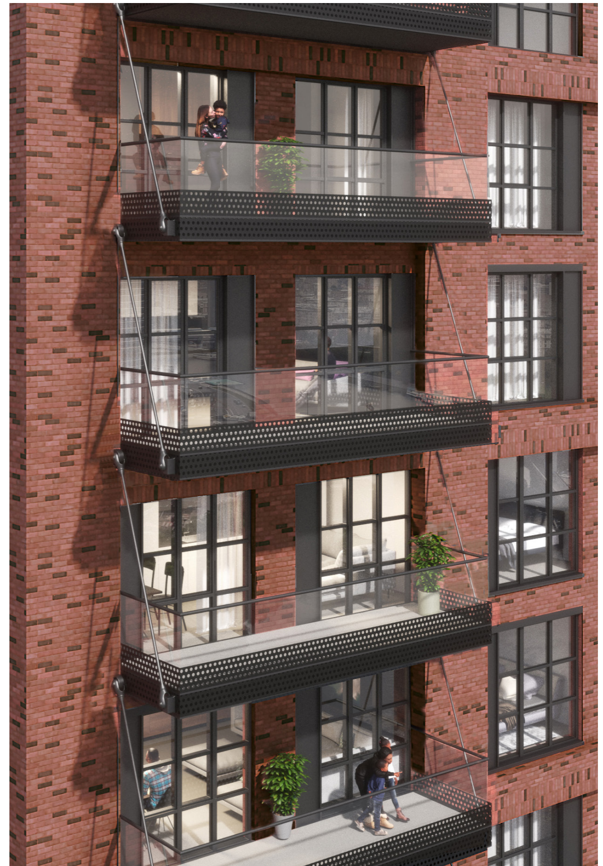
Blocks A and B - Balconies with perforated modesty panel
