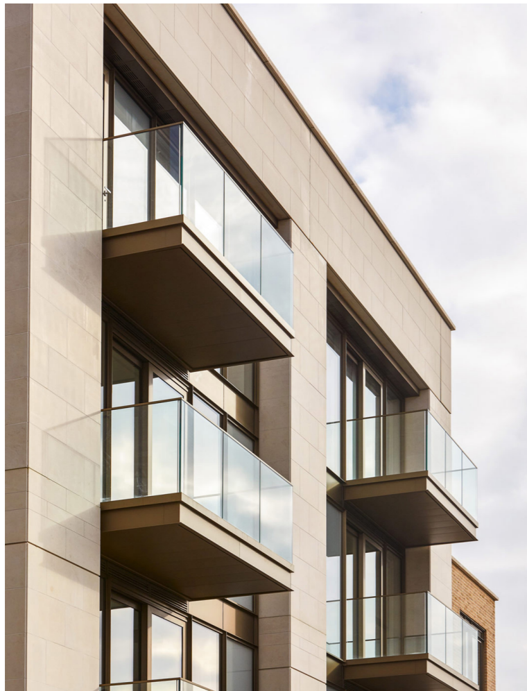
Lillie Square glazed balconies by JMP
