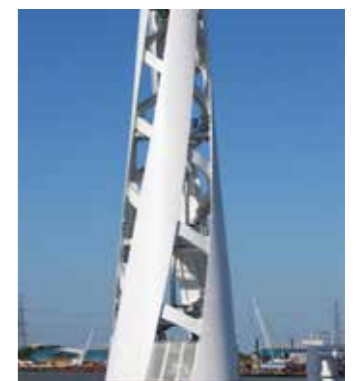
Cable car pylon
