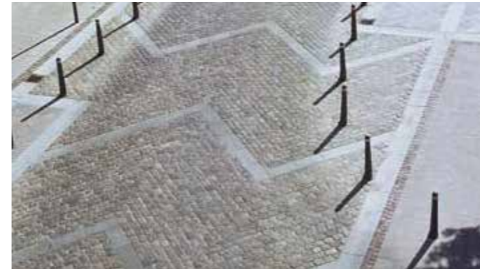
Patchwork of small unit paving
