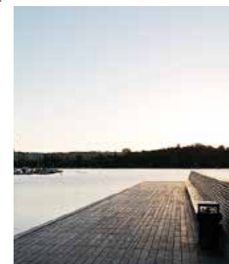
Decking to projecting jetties
