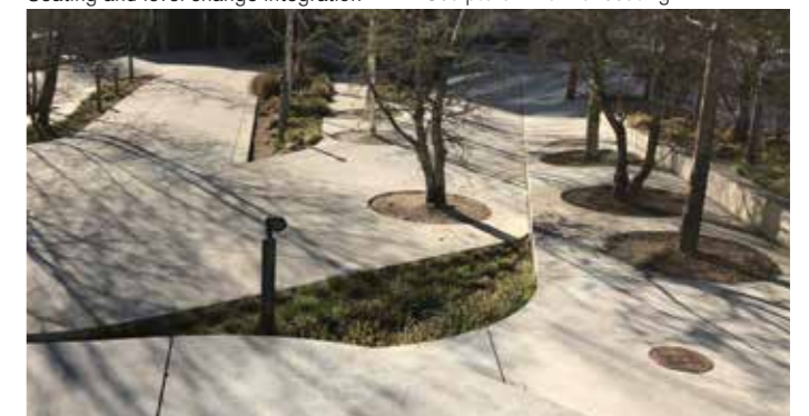
Planting bed and slope integration
