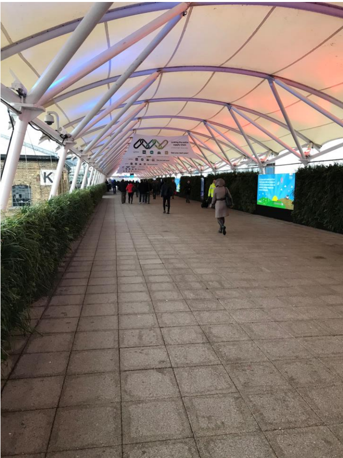
Covered walkway link to station entrances
