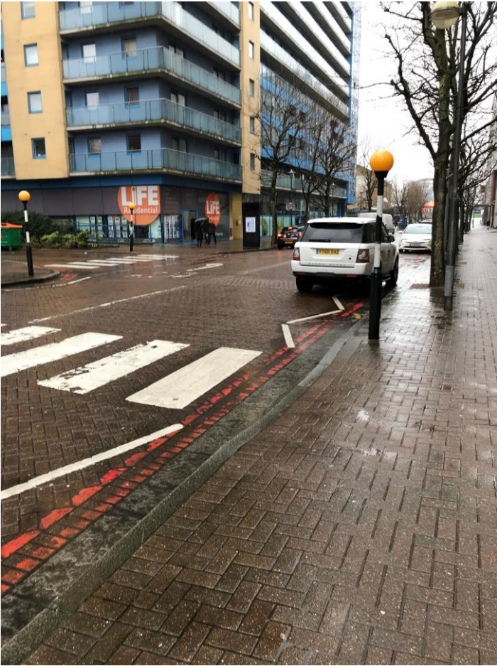
View east along Western Gateway
