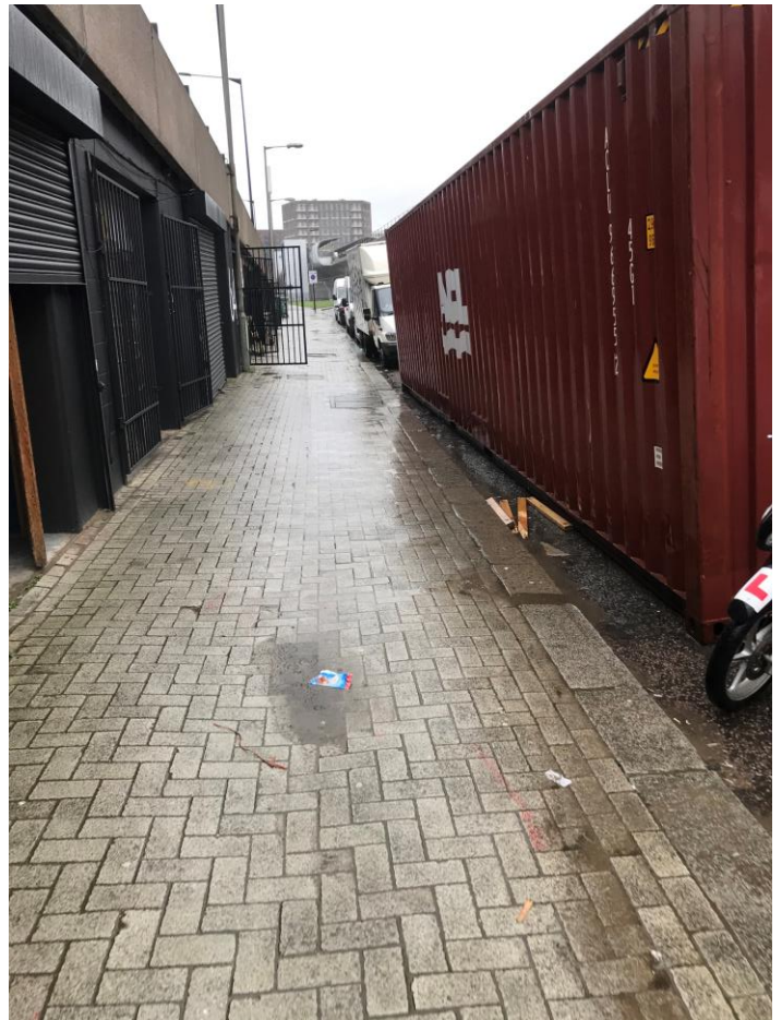
Footpath obstruction – outwards opening gates
