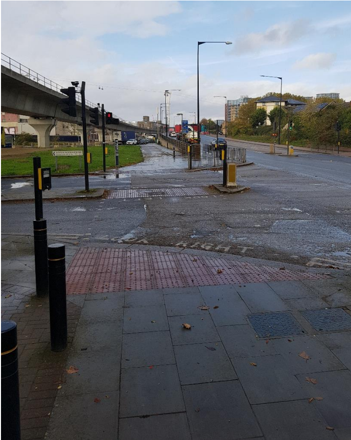
Figure 21. Pelican Crossing at A1020 Silvertown Way/North Woolwich Road junction.
