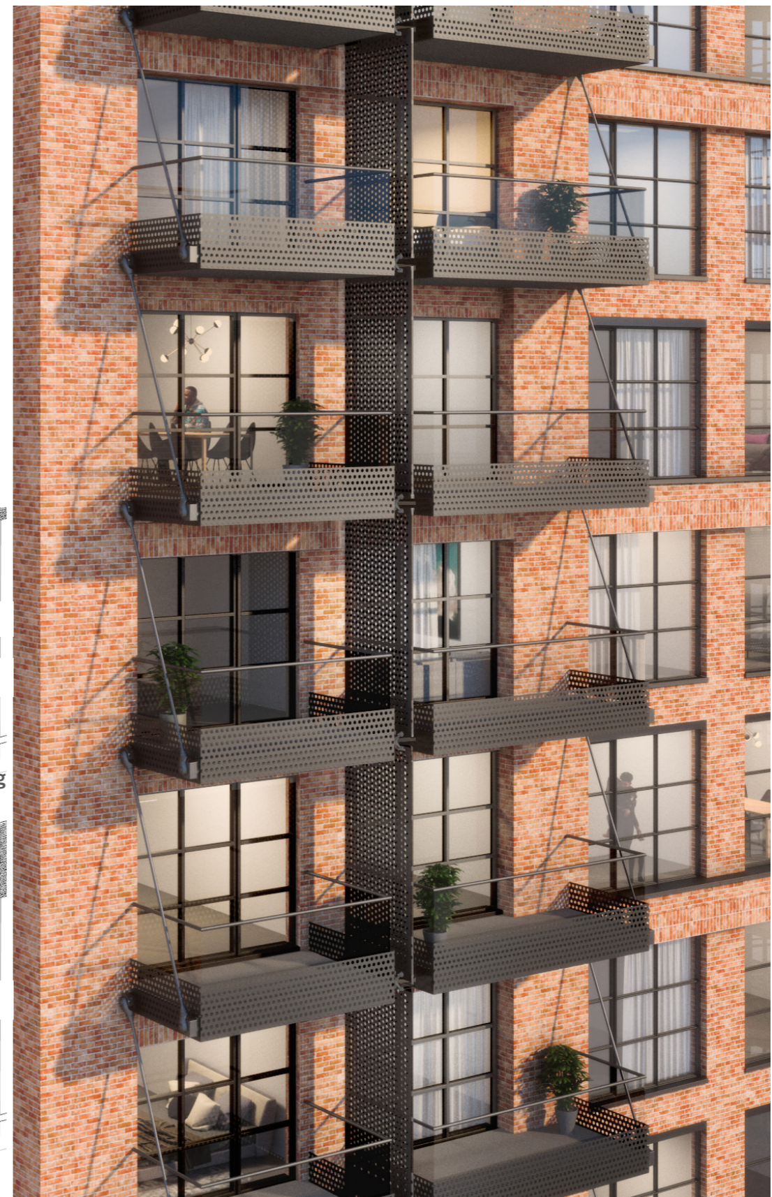
Block A - Balconies with perforated privacy screen
