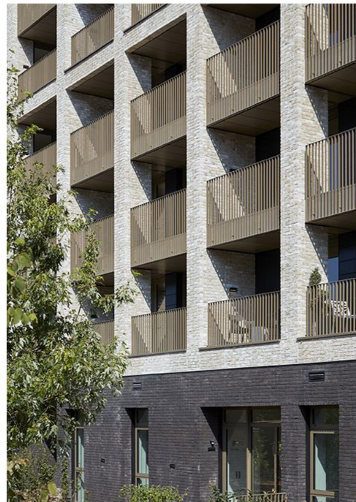
Inset metal balconies by AHMM
