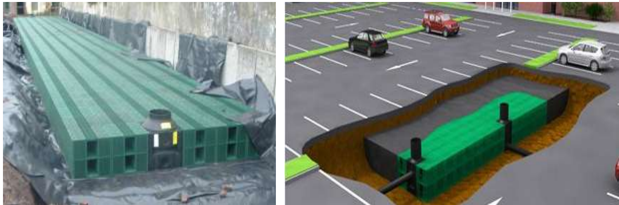
Figure 4: Typical Cellular Attenuation Tank
