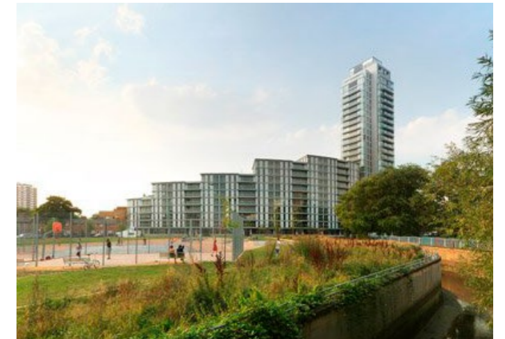
Seager Tower - John McAslan + Partners
