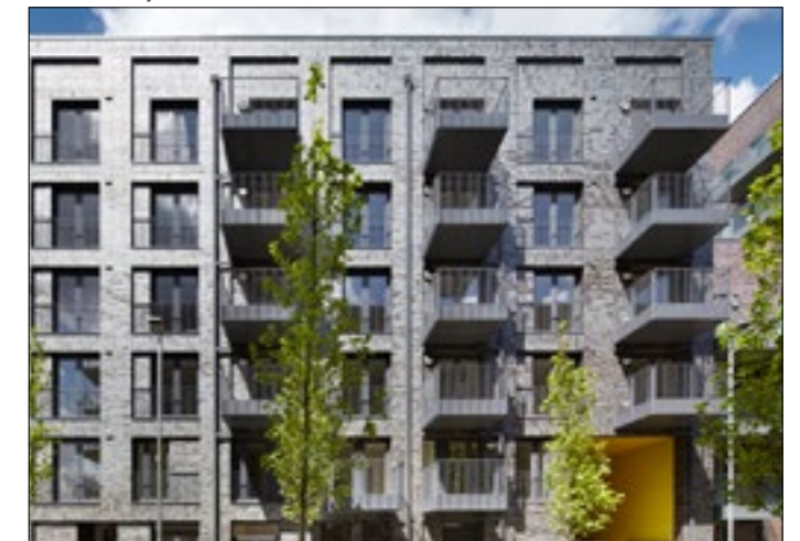
Mix of Projected Balconies and Juliet Balconies
