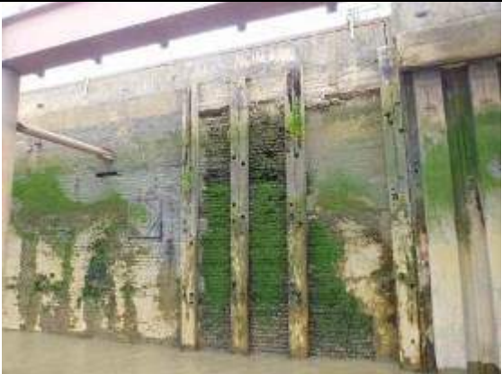
Figure 11 - View of older masonry and timber fenders at downstream end
