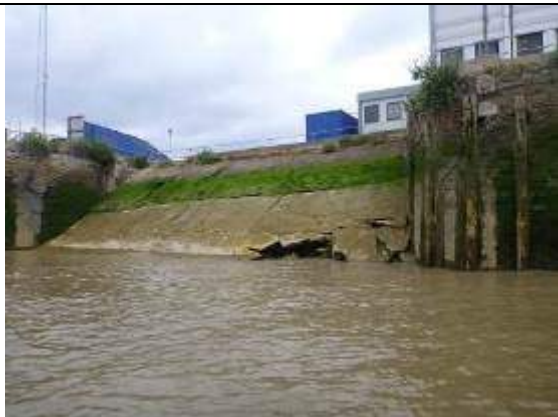
Figure 24 - Concrete apron and masonry abutments
