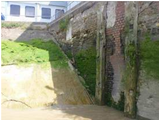
Figure 29 - Interface between masonry wall and masonry abutment. View of large sections of replacement masonry
