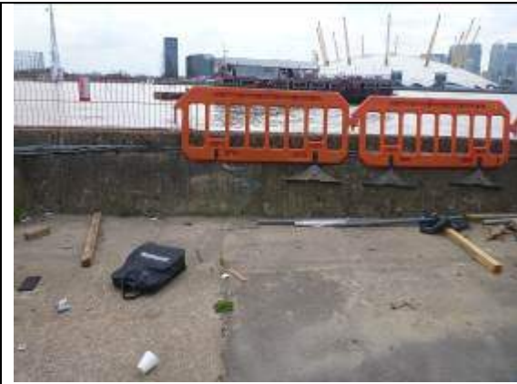
Figure 61 - Crack in river wall with resurfacing on the land directly behind the frontage
