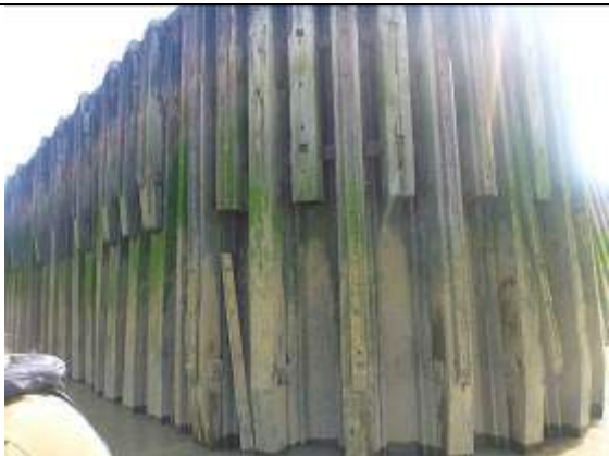
Figure 70 - Timber fenders on entrance to the dock
