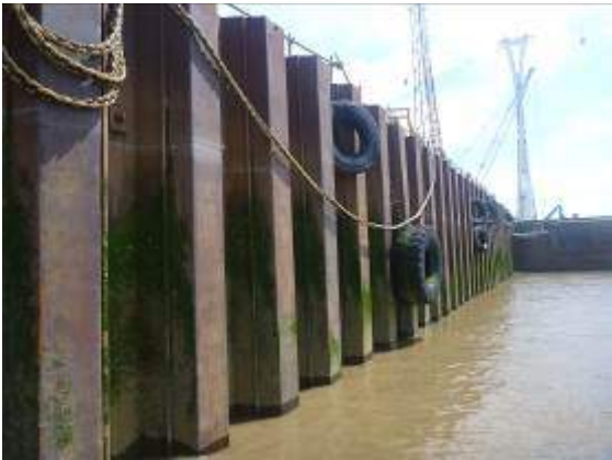
Figure 47 - Steel sheet pile wall
