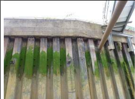
Figure 15 - Steel sheet pile with steel brace and concrete parapet
