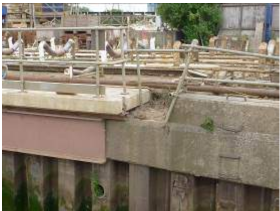
Figure 9 - Intersection between temporary structure and existing river wall
