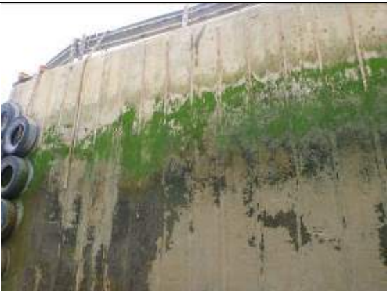
Figure 53 - Concrete abutments with steel railing reinforcement
