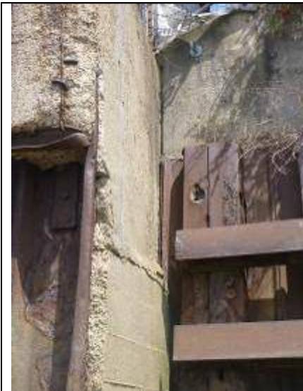
Figure 63 - Interface between steel sheet pile wall and adjacent upstream asset
