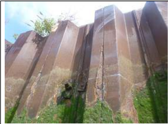
Figure 33 - Waling bolt on sheet pile wall
