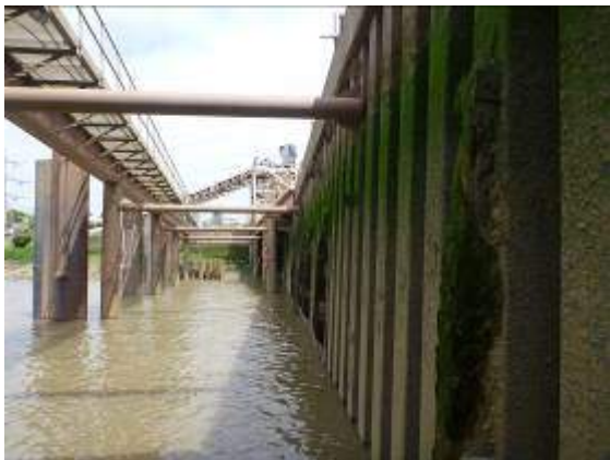
Figure 1 - Steel sheet pile wall with large diameter fender piles and rails for spoil transfer system
