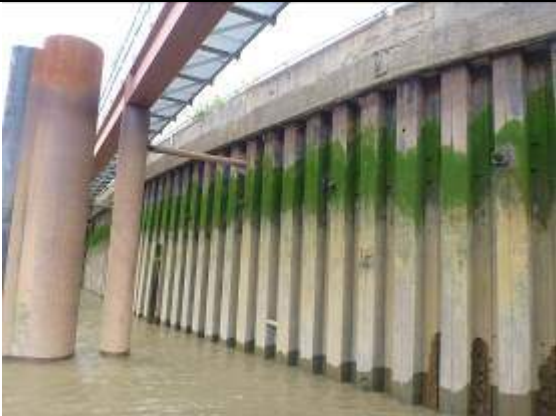
Figure 16 - Steel sheet pile with large diameter fender piles (left) and frame supporting rails for spoil hopper (behind)
