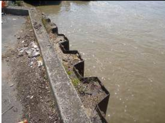
Figure 37 - Concrete backfill behind sheet piles and concrete parapet
