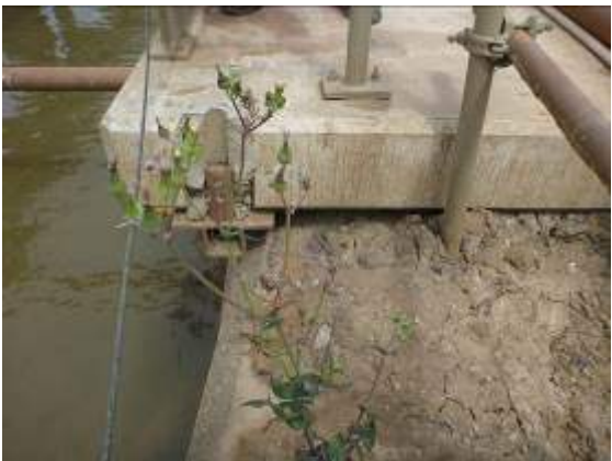
Figure 8 - Temporary structure covering ground at upstream extent of the frontage
