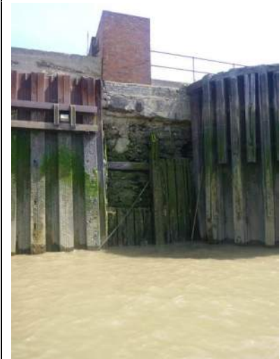
Figure 73 - Timber wall section at upstream extent of asset
