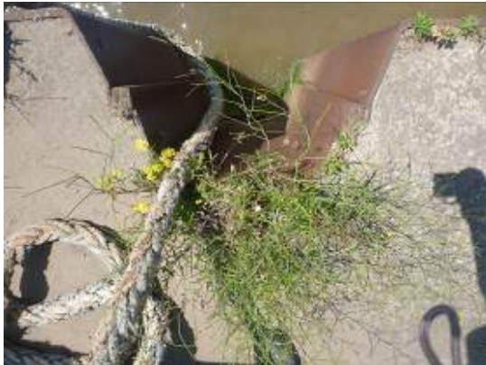
Figure 48 - Concrete back filling behind piles
