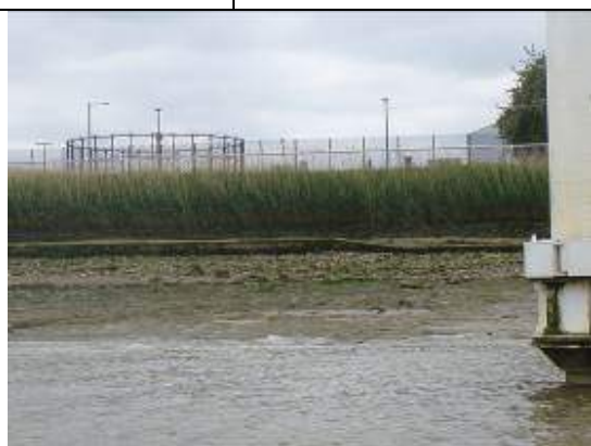
Figure 76 - Concrete wall is obstructed by reeds but gabion baskets at the toe are visible
