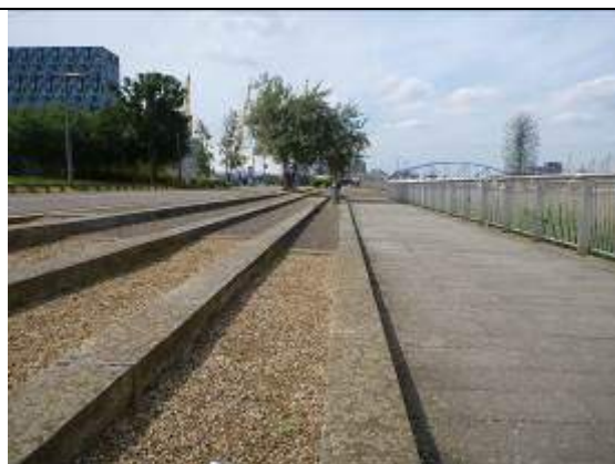
Figure 79 - Concrete steps up to second Thames Path - this is the flood defence level
