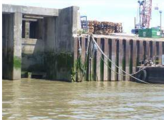
Figure 49 - Steel sheet pile wall and concrete Thames Water outfall
