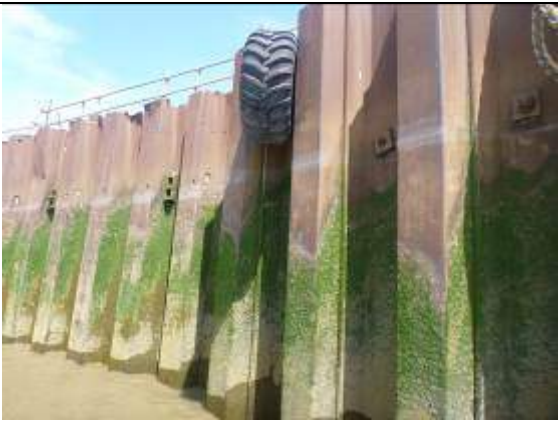
Figure 45 – View of upstream end of asset, showing how the piles have been driven in front of existing frontage
