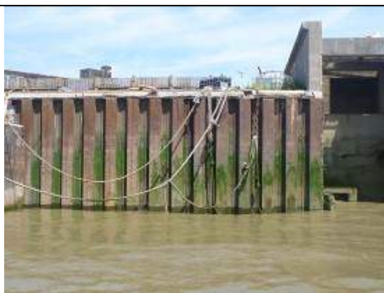
Figure 50 - Steel sheet pile wall adjacent to Thames Water outfall
