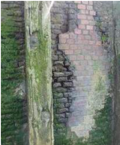
Figure 27 - Repaired section of masonry wall
