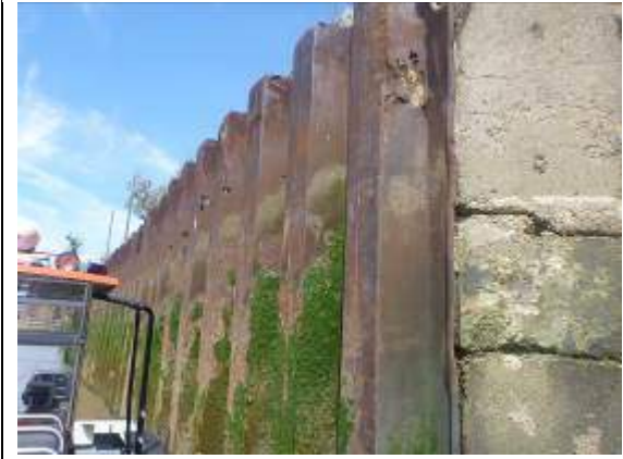
Figure 35 – View of steel sheet pile wall and concrete interface
