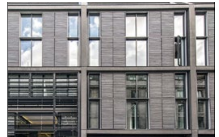
Regular window pattern and shape, grey brick panels
