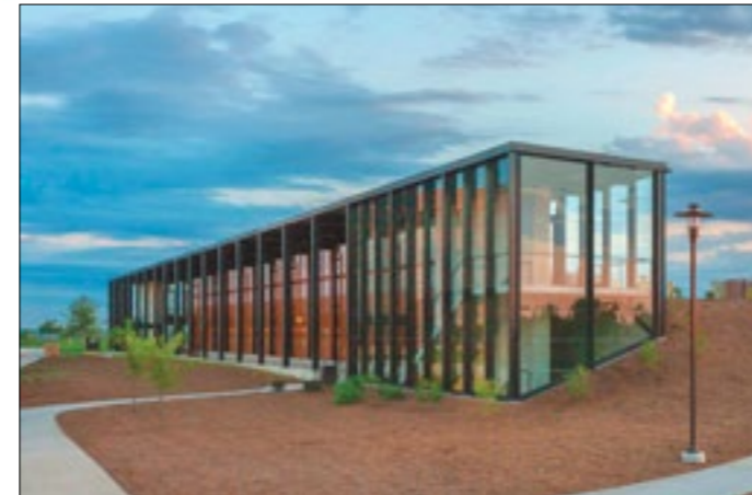
Metal and concrete emphasize an industrial look and feel
