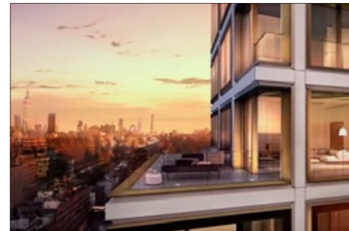
Expressed precast concrete and metal frame
