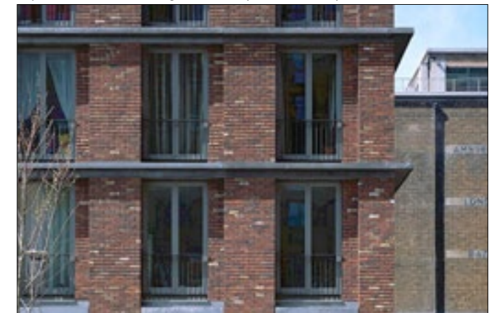
Expressed precast concrete and brick, Juliet metal balconies
