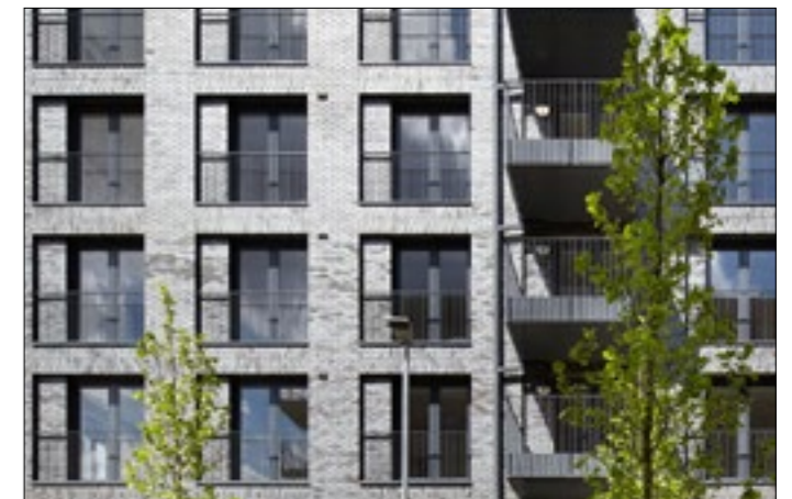
Regular window pattern and shape, light grey materiality, varying balconies
