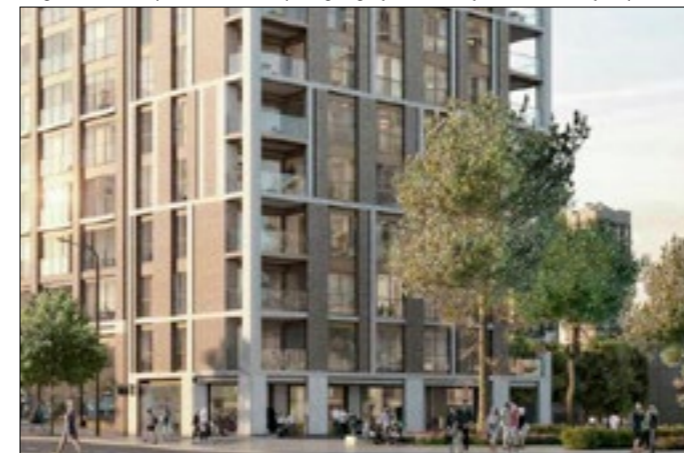
Masonry frames, precast concrete and brick, set-back balconies
