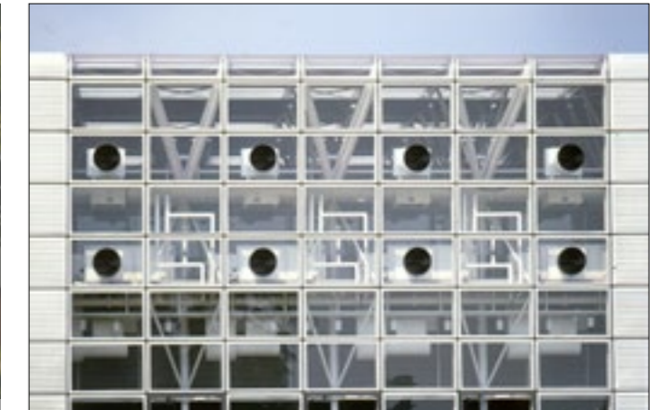
Large span structure allowing daylight through various solid and transparent panels
