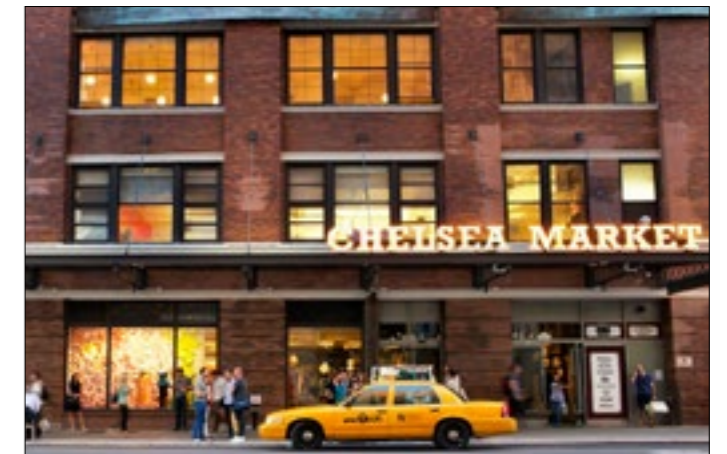
Expressed brick frames, regular window pattern and shape
