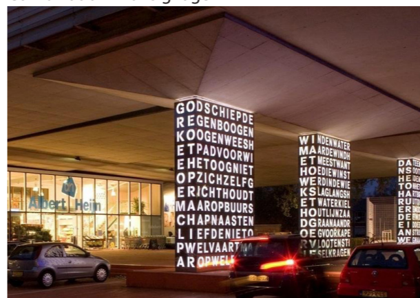
Dressing the viaduct
