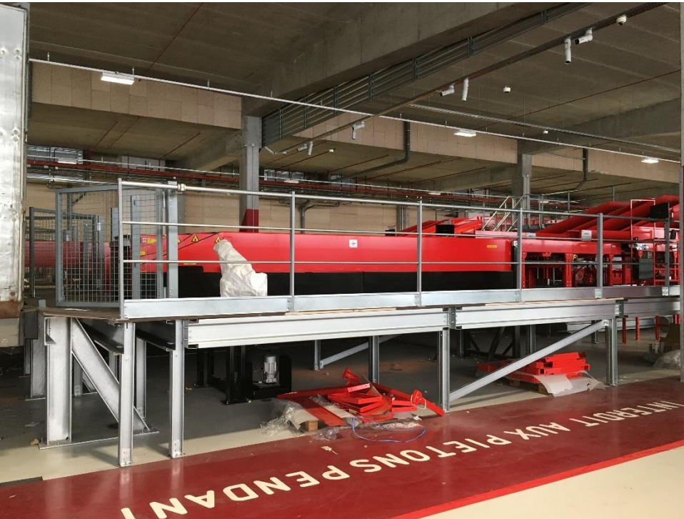
Image 3: La Chappelle International – DPD operating inside the building
