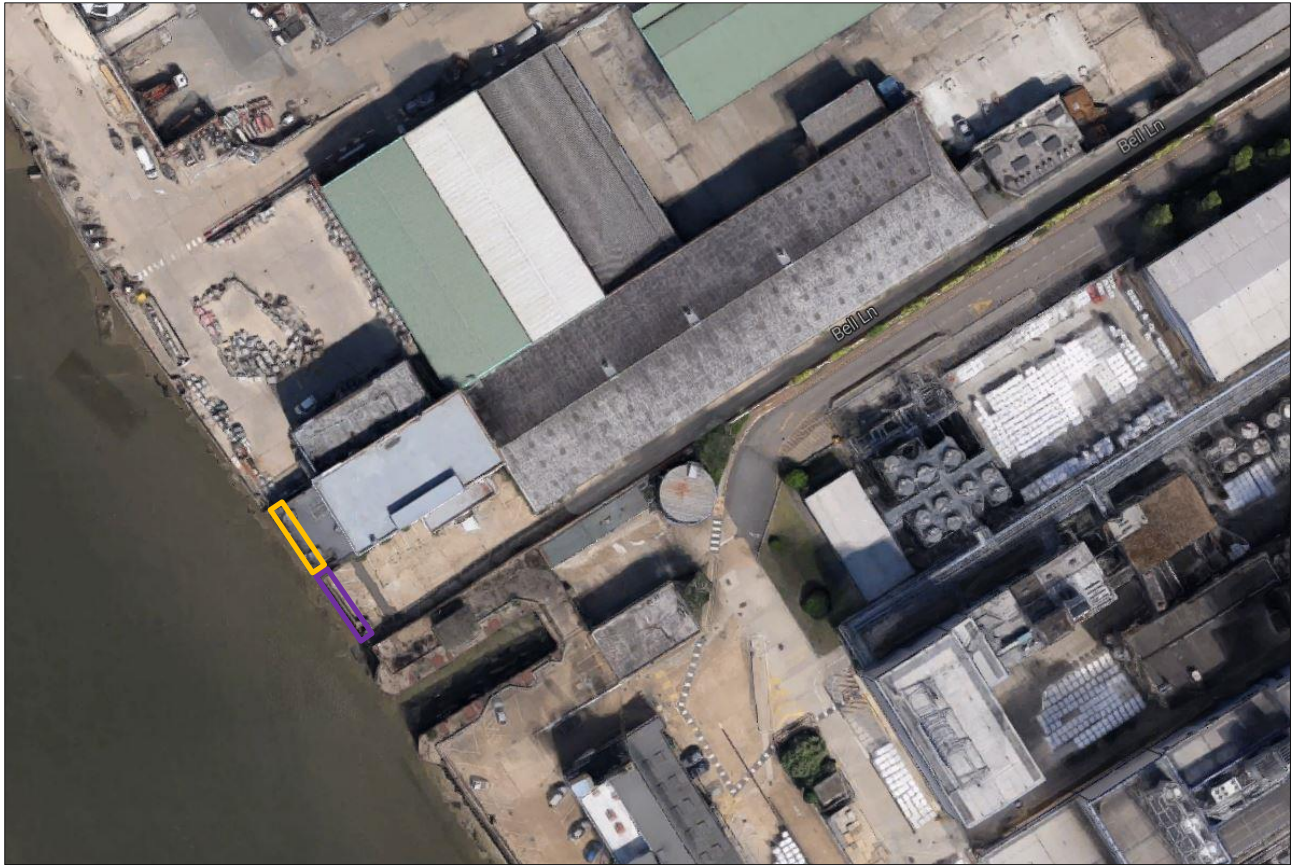
Figure 2.1: Aerial view of Dohm Wharf showing inspection areas
