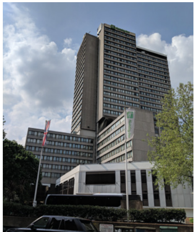
Existing Building - View from Courtfield Road
