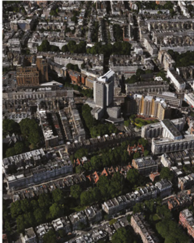
North view of the building from the south. Quantifying how the character and articulation of the existing building does not respond to the materiality and richness of the neighbouring context.
