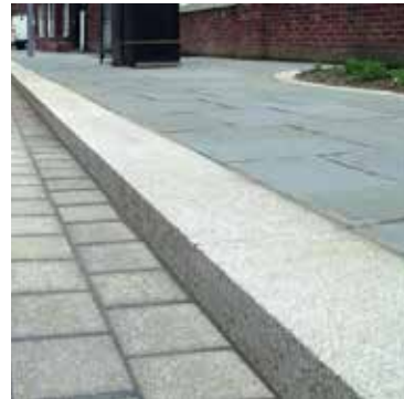
Edge Type 02 Granite Kerb Supplier: Marshalls
