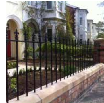
Railing to low brick wall (brick to match arch. specification to Courtfield Road elevation) Height: 1.8m (total) 600mm wall 1200mm railing
