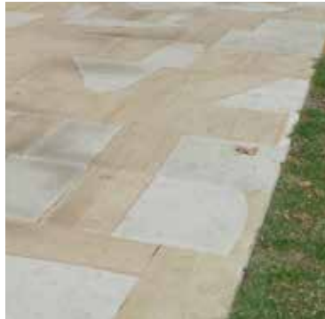
Surface Type 01 Yorkstone 'Scoutmoor' Paving Supplier: Marshalls Size: 600x random lengths x63mm Finish: Diamond sawn
