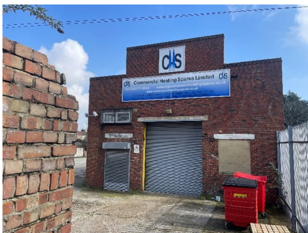
Figure 3-2 Brickwork Facade – 4 Sedgemere Road
