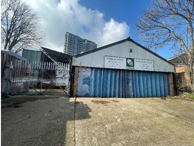
Figure 2-11 8 Sedgemere Road (Eastern Elevation)
