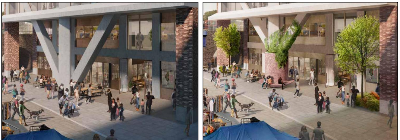
Figures 7a and 7b – Originally proposed (left) and currently proposed (right) structural cross bracing [Image from DAS addendum September 2020].
