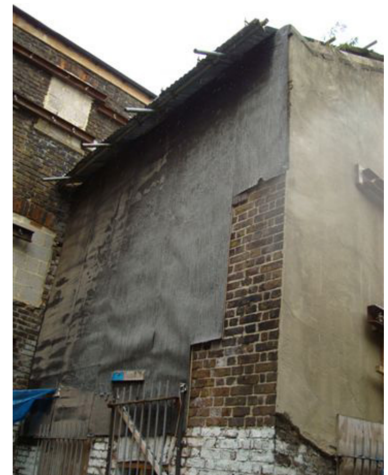
Existing Cottages. Rear elevation
