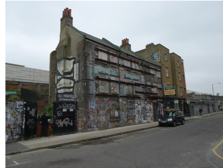
Existing Cottages. Sclater street view
