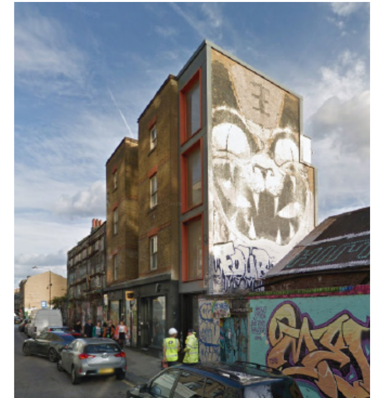
Photograph of existing unsympathetic side extension on Sclater Street
