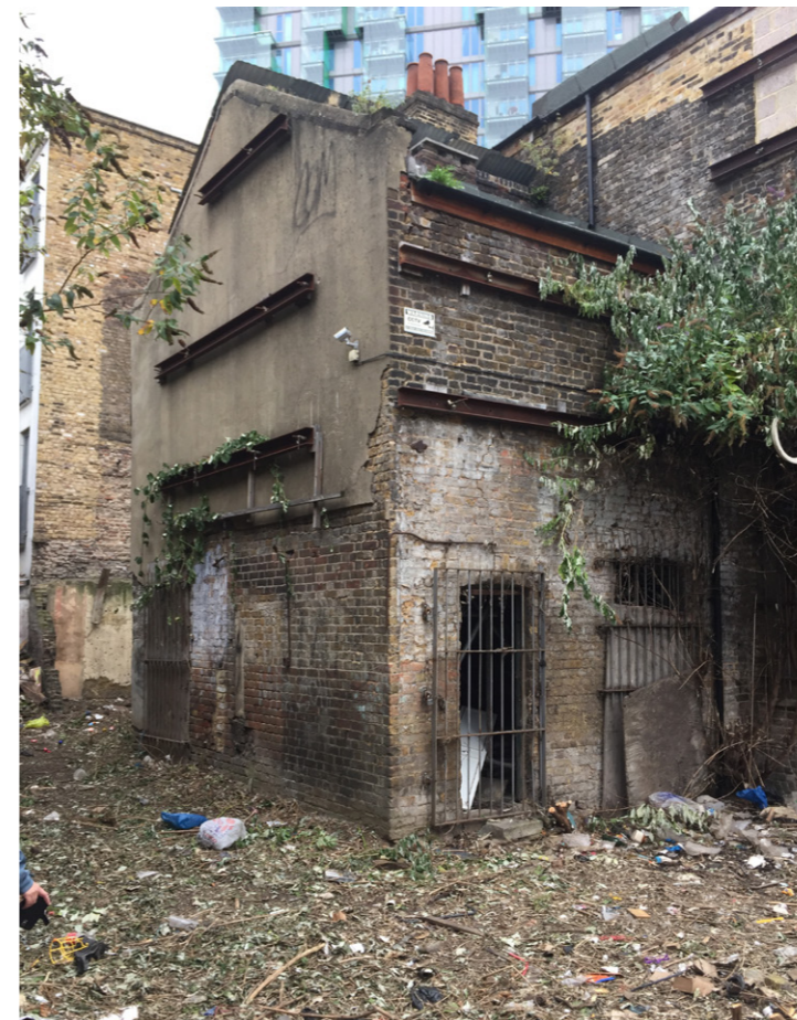
Existing Cottages. Rear elevation
