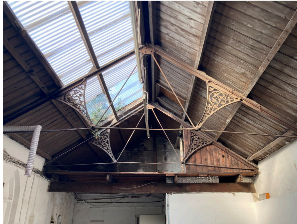
Mission Chapel roof structure, to be retained
