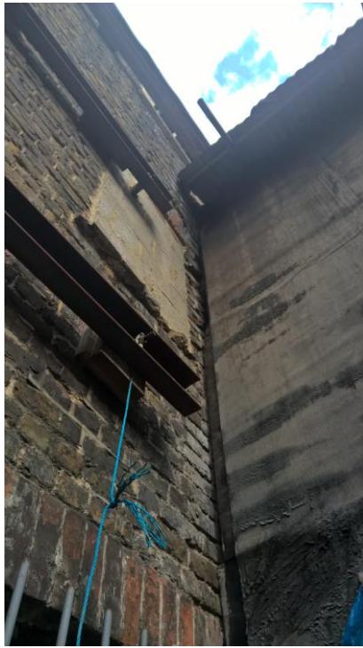
Junction of rear wall to west wall of rear addition to Number 72 Sclater Street
