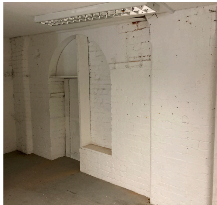
Station Wall inside the Mission Hall
