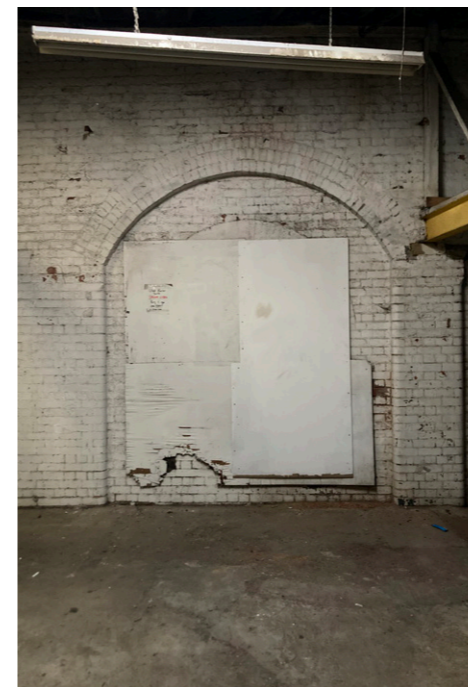
Station Wall inside the Mission Hall western extension
