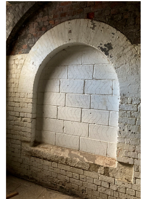
Station Wall inside the Victorian Building
