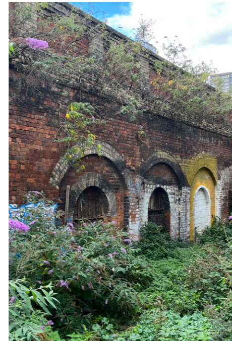
Station Wall behind the Weavers Cottages
