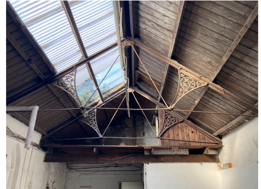
Mission Hall - Photograph of existing iron roof structure
