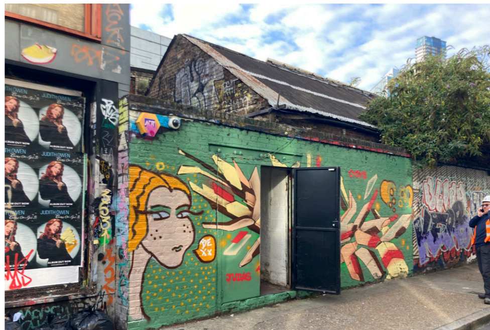
Photograph of the existing 20th century wall screening the Mission Hall off from Sclater street
