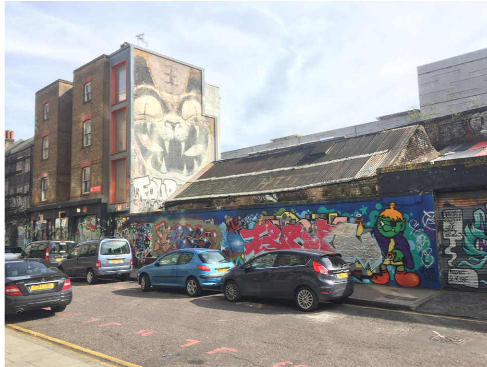
Photograph of the existing 20th century wall screening the Mission Hall off from Sclater street
