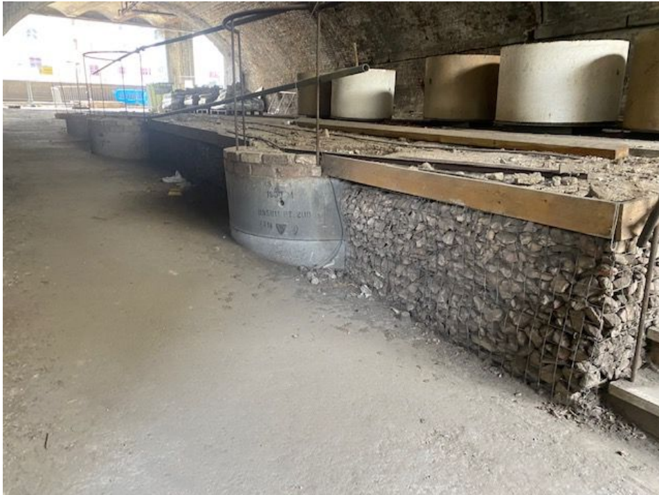
Old railway in eastern arches built up with gravel fill
