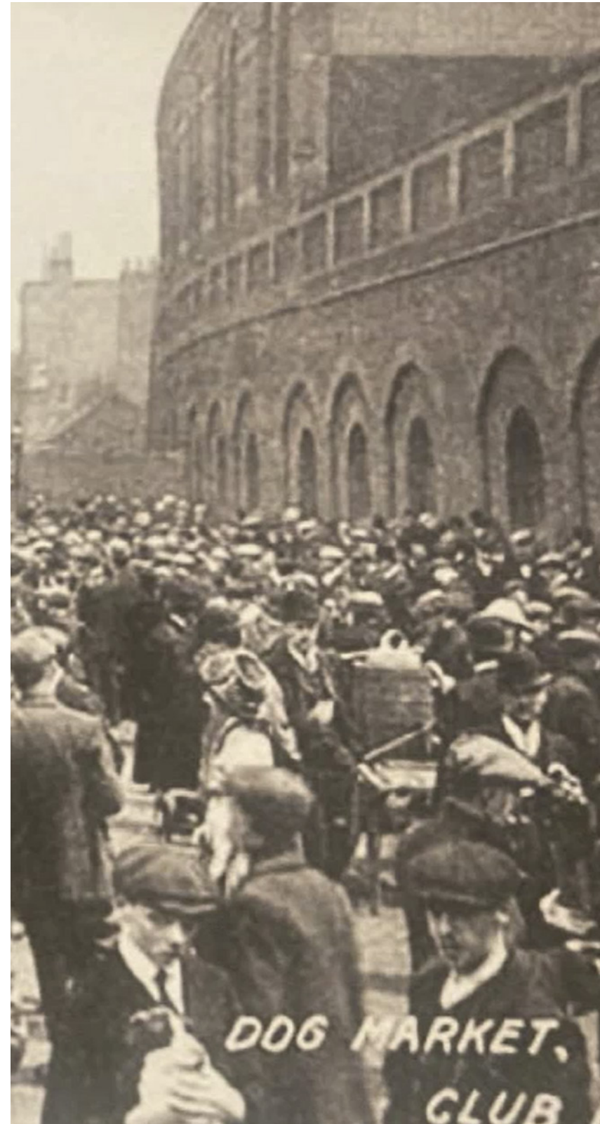
Existing Historical boundary wall with Arches on Sclater Street
