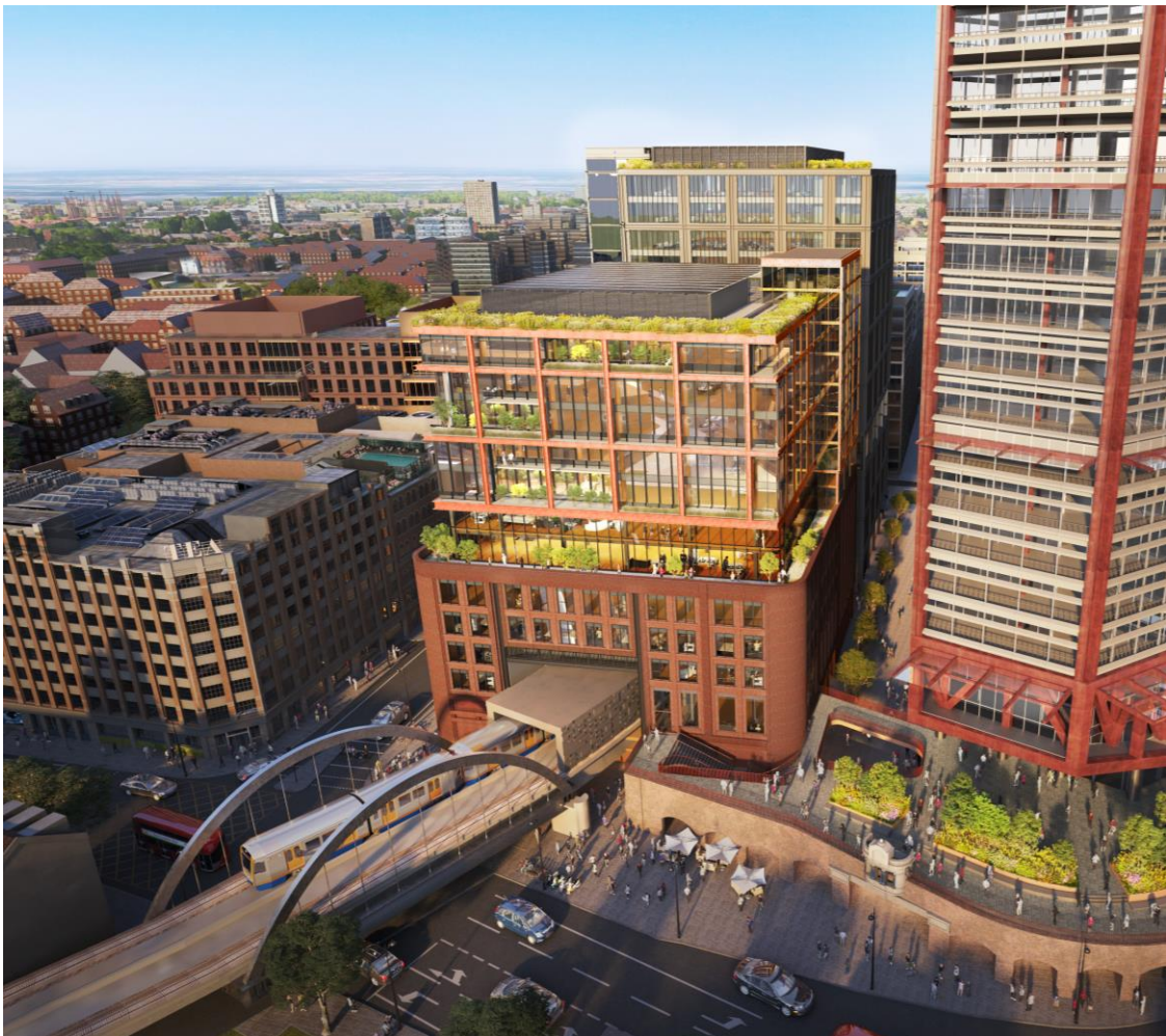
Figure 1.2 Visualisation of Plot 1, showing how the London Overground Line runs through the building.
