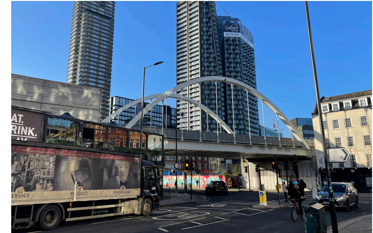
The Overground Bridge extending over Shoreditch High Street
