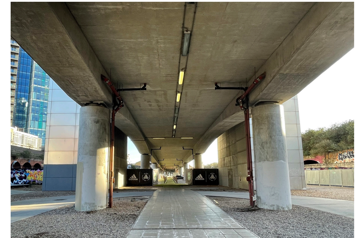
The Overground Supports at ground level
