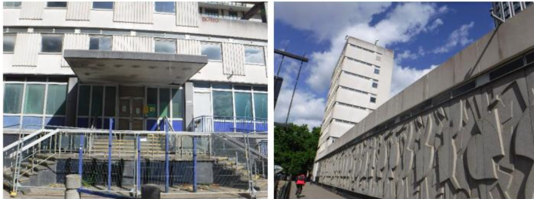
GENERAL VIEWS THROUGHOUT
