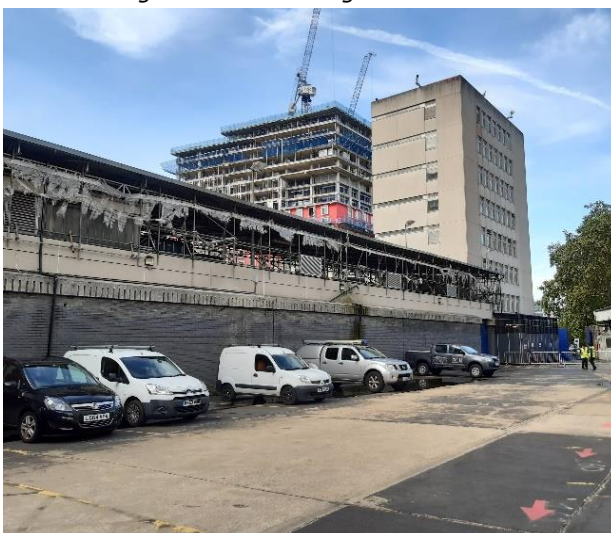
Surfaced Car Parking Area and Link Block
