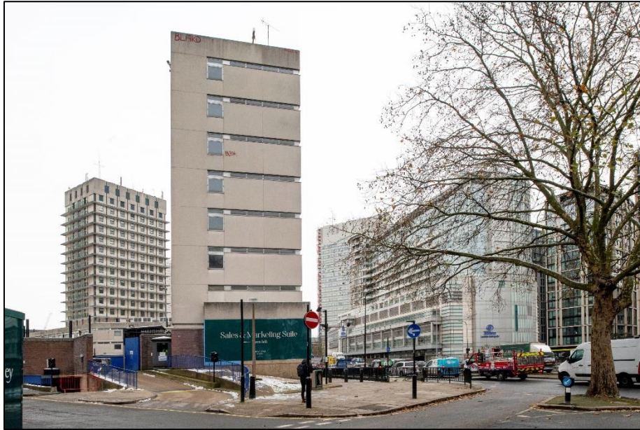
Fig 108 The west elevation of the eight-storey tower, looking east (A. Chopping) 035322004
