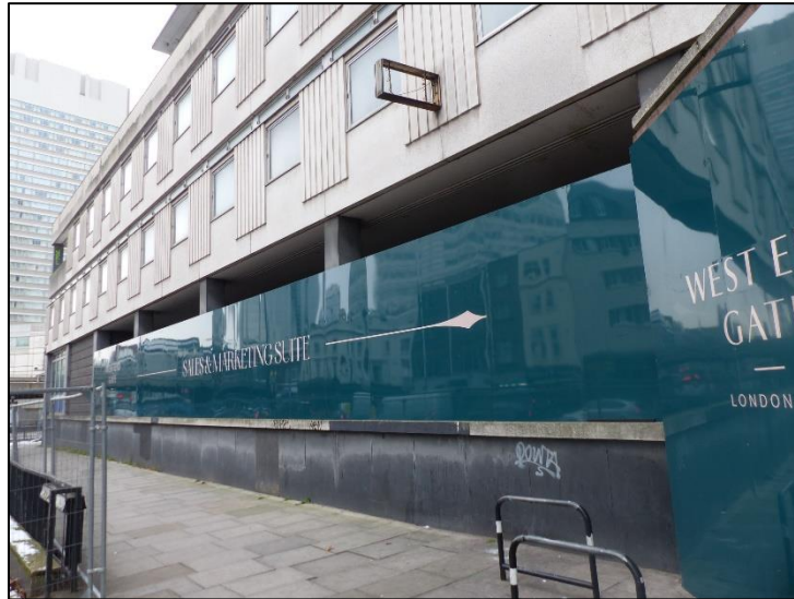
Fig 23 The north-east facing elevation to the pentagonal range P1330194
