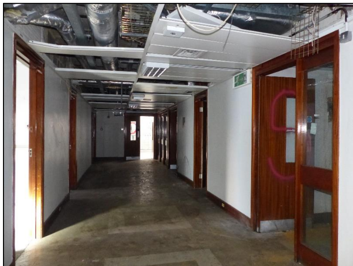
Fig 77 First floor corridor looking south-west P1400256
