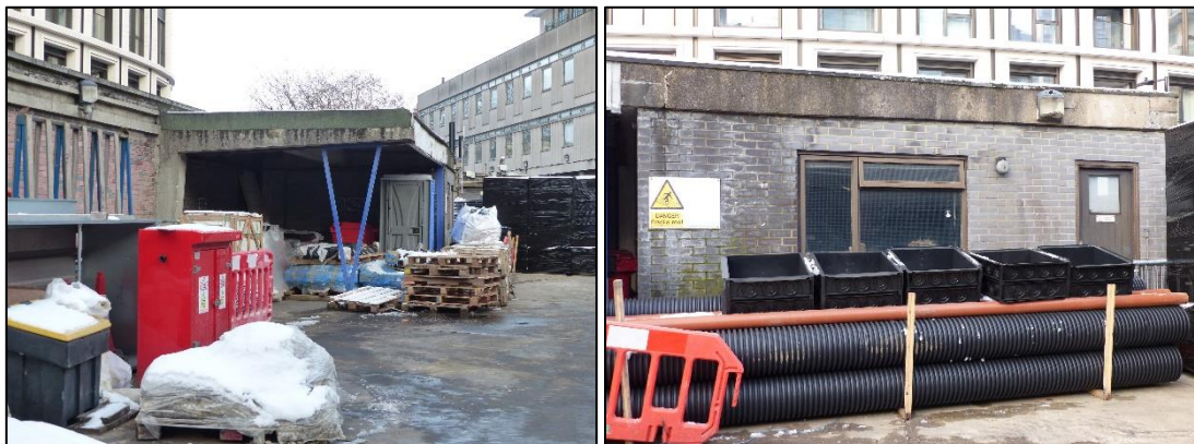
Fig 104 Two examples of the sentry buildings within the yard, looking east (left) and north (right) P1400310 & P1400311
