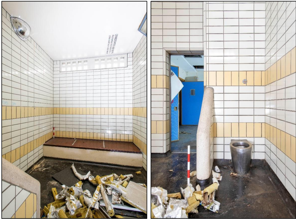
Fig 63 An example of a tiled holding cell, looking north 035322013, 035322014
