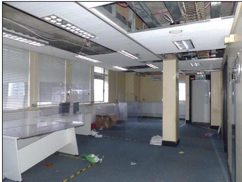
Fig 125 A general view of the fourth floor demonstrating the more open floorplan, looking east P1400345
