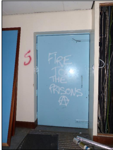
Fig 73 The sealed access door to the eight-storey office block, looking west P1400202
