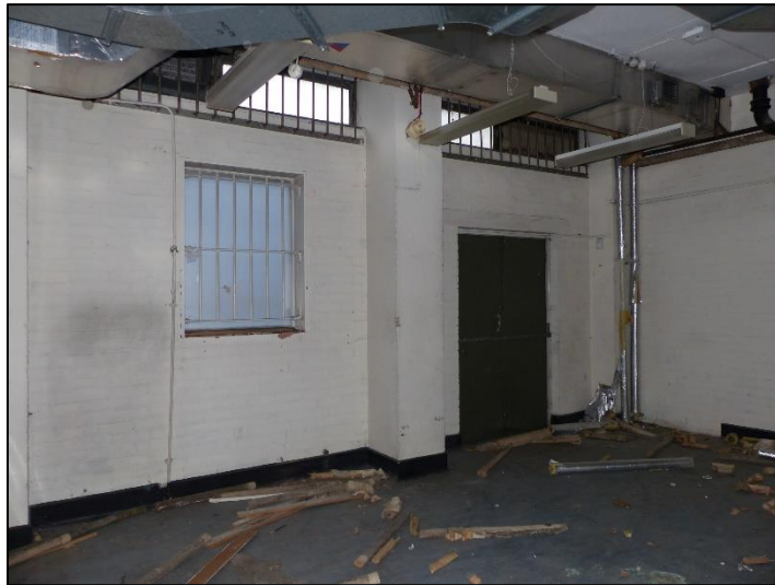
Fig 76 An example of ground floor storage areas, looking north-west P1400230
