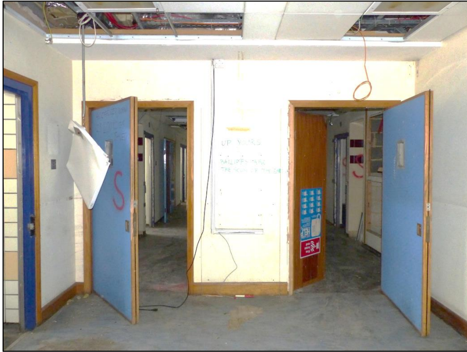
Fig 56 The custody office access to the cell block, looking west P1400156
