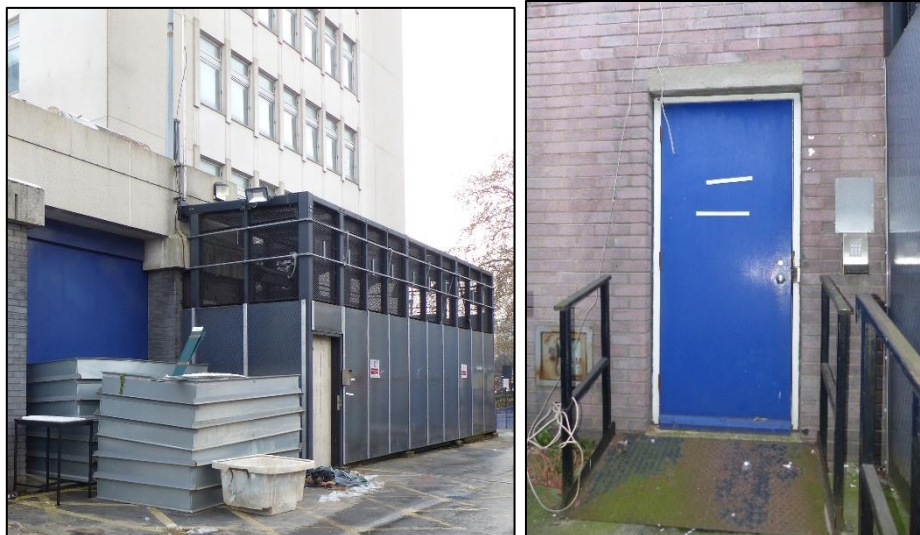
Fig 107 The caged exercise area, looking south-west P1400305 and the access door to the building, looking south P1400326
