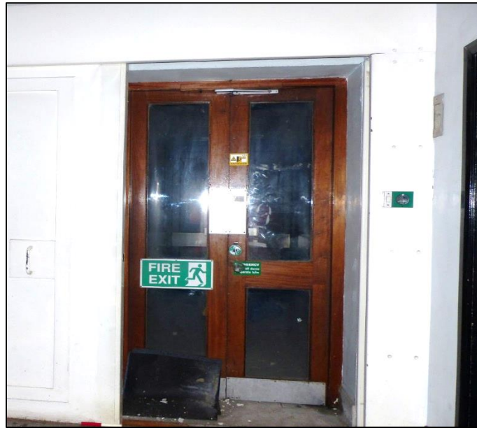
Fig 112 The glazed doors behind the sliding security door, looking west P1400334
