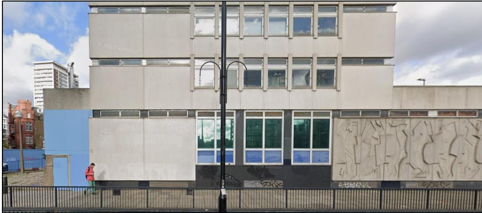
Fig 105 The south elevation of the eight-storey tower, looking north (Google Earth, 2022) Picture1.png
