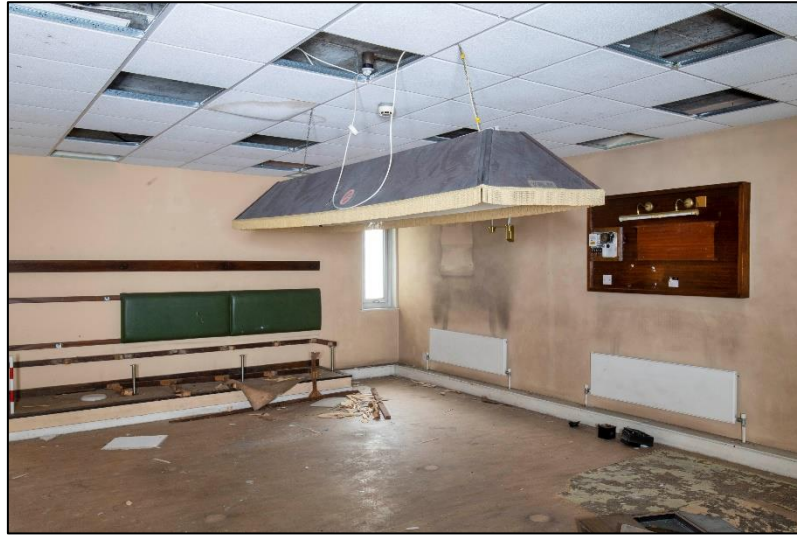
Fig 86 The billiards room to the third floor, looking south-east (A. Chopping) 035322032
