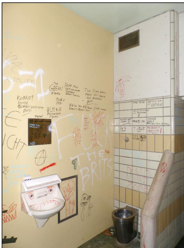
Fig 67 View of facilities in the high security cells, looking south-west P1400189
