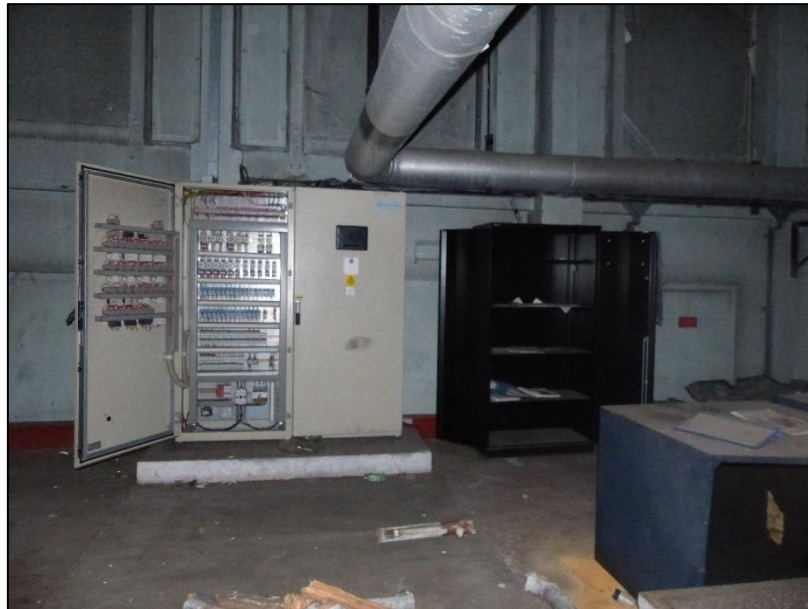
Fig 93 The fifteenth floor, looking north P1330213
