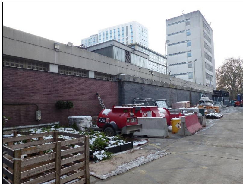
Fig 97 The north elevations of the single storey range containing the cells, looking south-west P1400291
