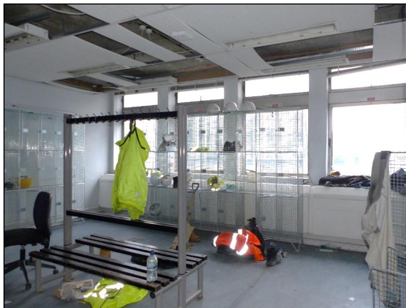
Fig 121 A typical room in the eight-storey tower block, looking south-east P1400338
