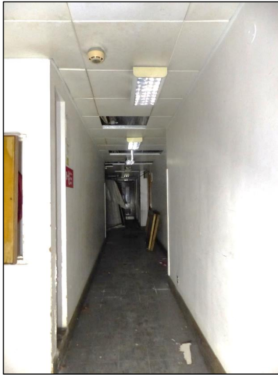
Fig 36 The corridor leading to the former Sargent's room, looking south-west P1330251
