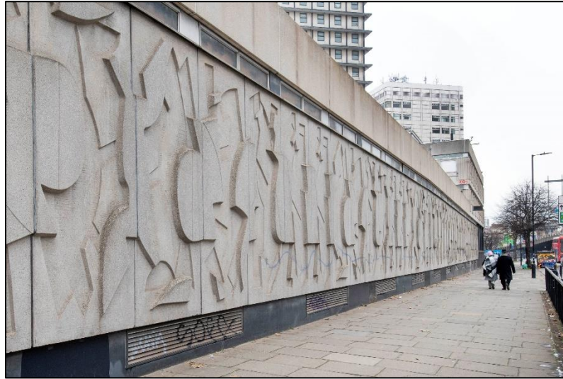
Fig 96 the south elevation of the single storey range, looking east (A. Chopping) 035322033.jpg
