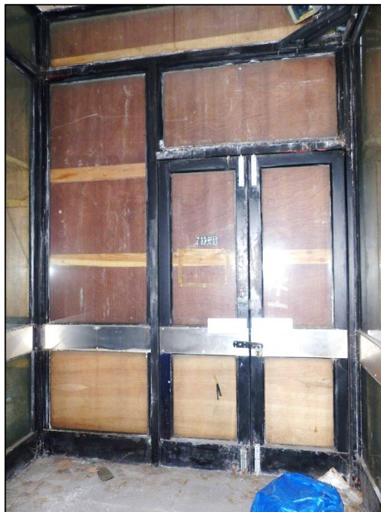
Fig 111 The glazed metal doors from Newcastle Place, looking west P1400333
