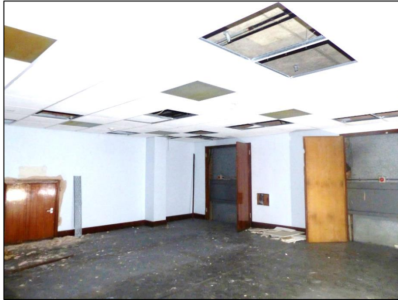
Fig 38 The former Sargent's room in the basement, looking north-west P1330247
