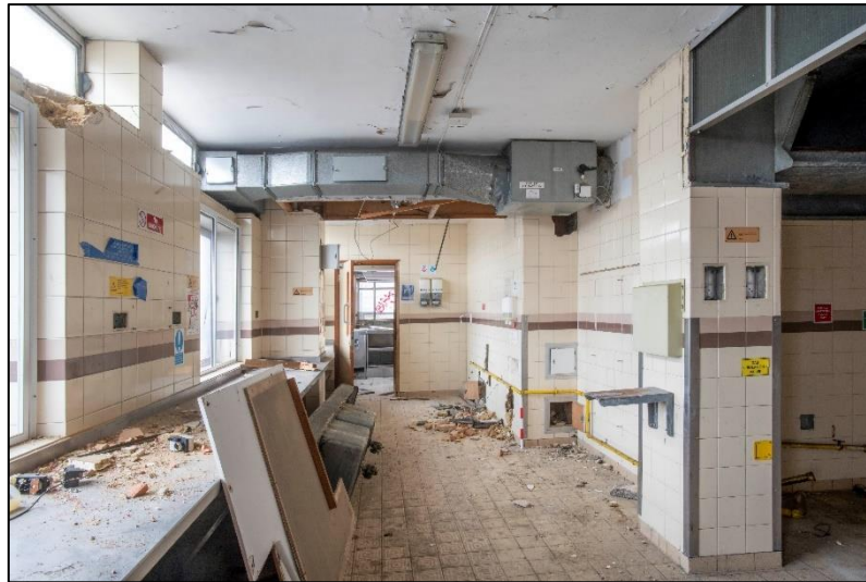
Fig 82 A general view of the kitchen, looking south-east (A. Chopping) 035322025
