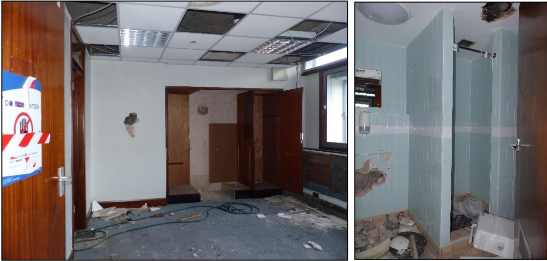
Fig 78 The Sargent's room, first floor looking north-east P1400257 and south-west P1400258
