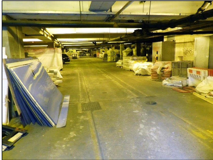
Fig 34 General view of the parking garage, looking east P1330287
