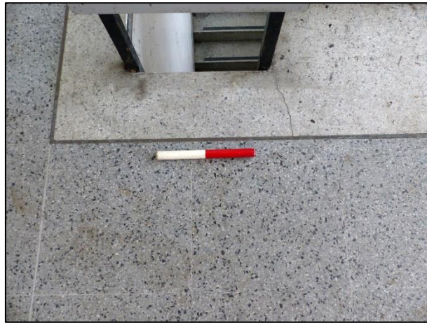
Fig 50 Detail to the terrazzo flooring, looking west P1400287
