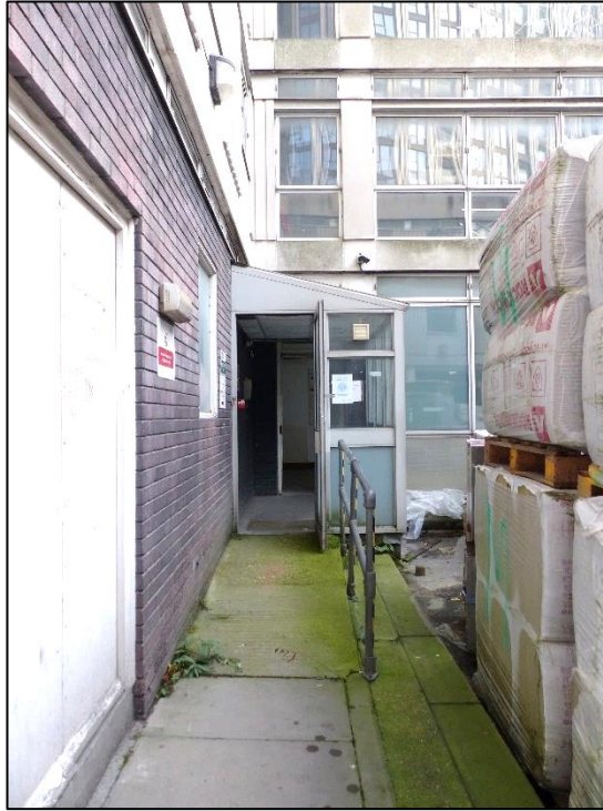
Fig 32 Access to the ground floor of the pentagon from the north-east wall of the yard, looking south P1400317
