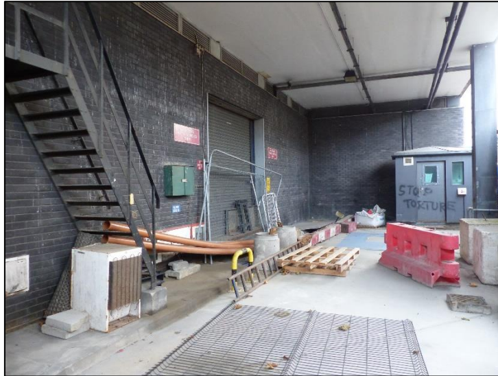
Fig 25 The former police and visitor parking area to the north-west side of the ground floor, looking west P1400295
