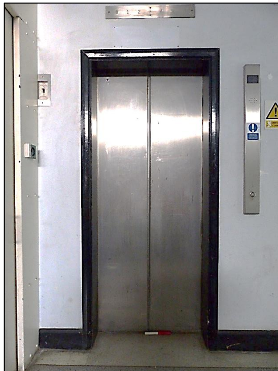
Fig 115 The lift in the ground floor entrance hall, looking north P1400330
