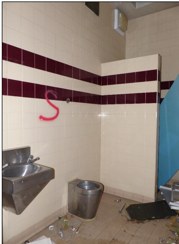
Fig 70 Shared toilet and shower to high security section, looking north-west P1400199
