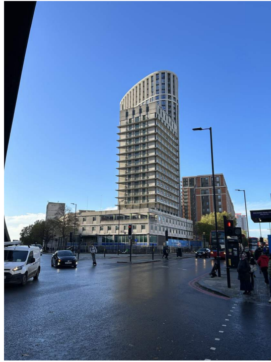
View 4 - View of site from below flyover
