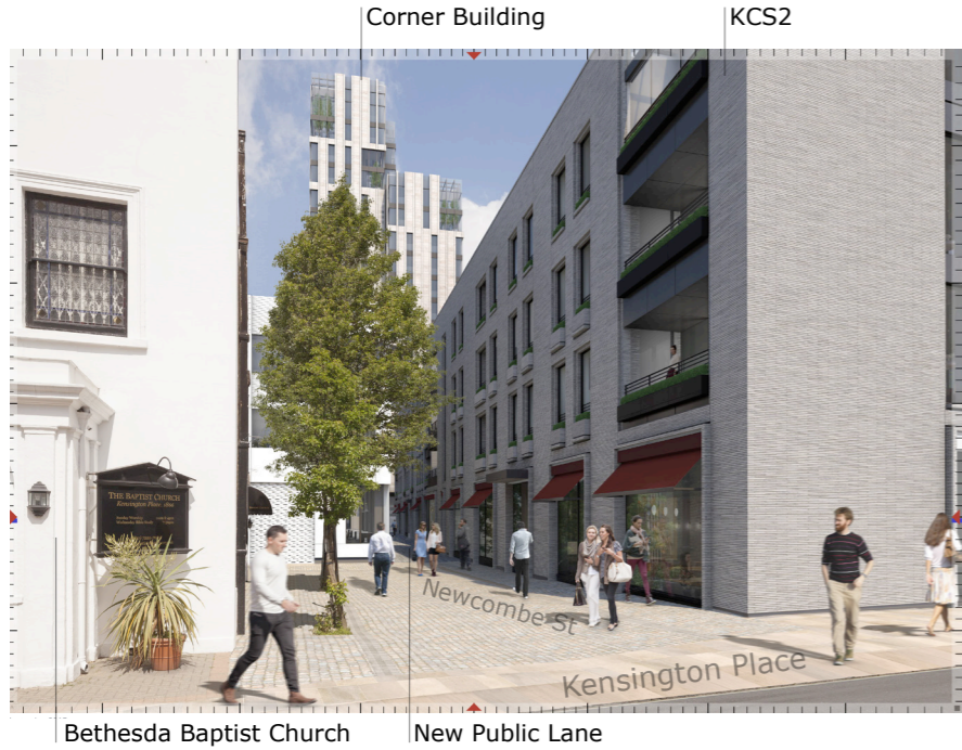
GLA Call In July 2018 - Proposed View 29(L1). Kensington Place - Looking North along Newcombe Street (Miller Hare verified view)
