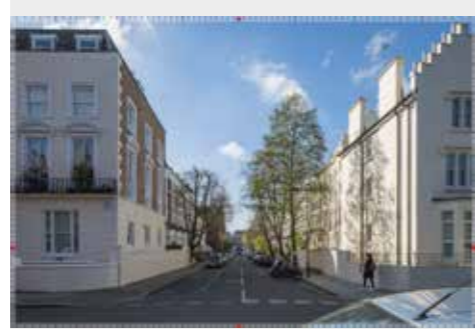
A2 | view A2(A2) | Talbot Road, looking south along Moorhouse Road
