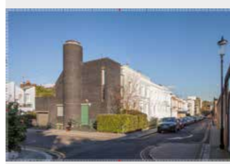
24 | view 24(L7) | Kensington Place - Junction with Hillgate Place
