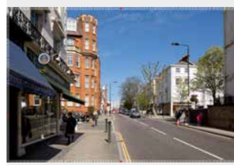
2 | view 2(1) | Kensington Church Street - South of Gloucester Walk | Spring
