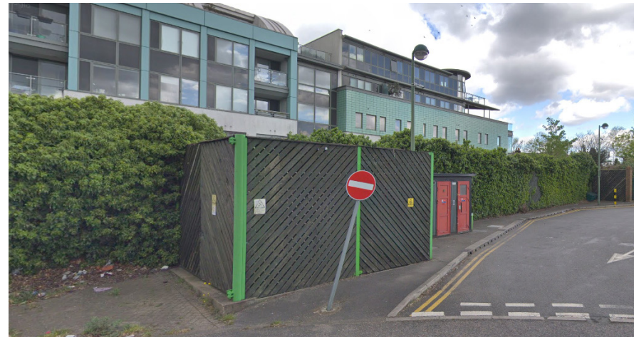
EXISTING SUB STATION ENCLOSURE
