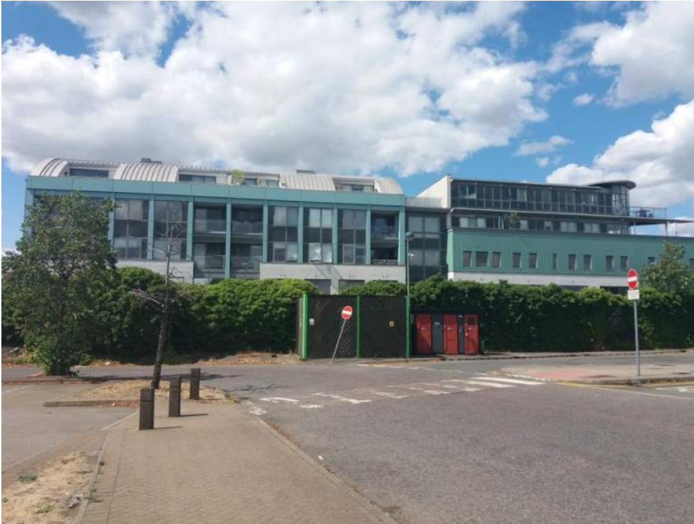
Photo 3: Looking west from site access towards electrical substation
