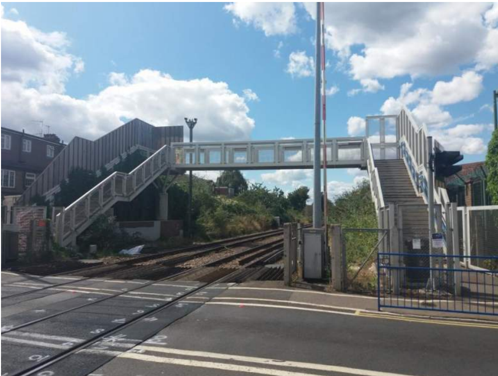
Photo 18: Footbridge adjacent to the south-east of the site
