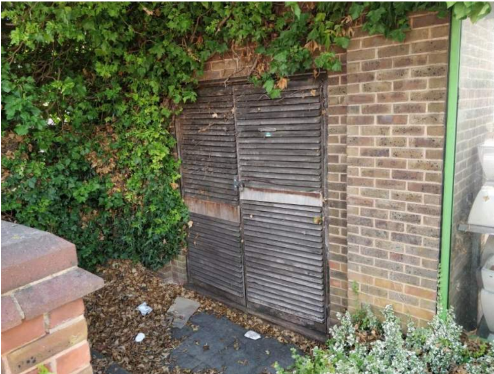
Photo 7: Brick structure assumed to be occupied by Southern Gas Network
