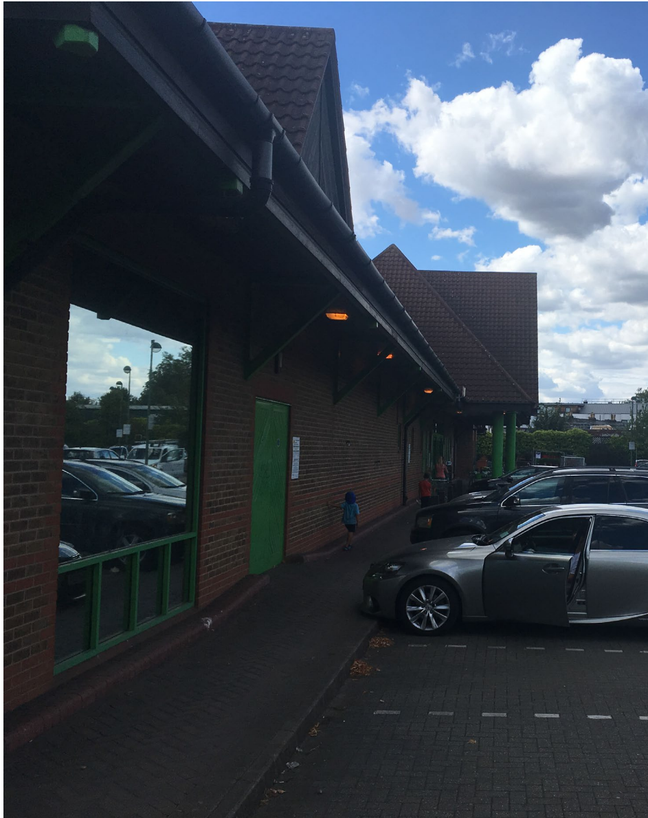
Photograph 3.4: View of the building from the front, facing north (view east).
