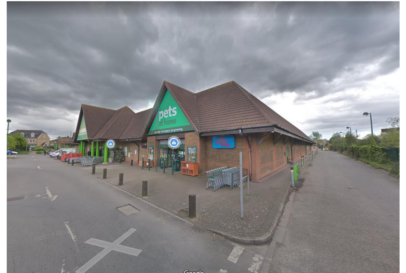
Figure 6: Existing Site structures: Homebase store and hardstanding (image from Google Streetview).
