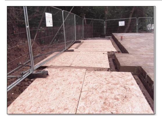
Installing heavy-duty OSB boarding over a depth (min. 50mm) of sharp sand and/or wood chip between the tree protection fencing and the foundation line of new development is effective in protecting roots, which grow in the soil beyond the position of the fencing.
