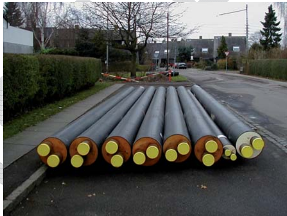
Figure 13: Twin Pipes for District Heating (image courtesy of Ramboll)
