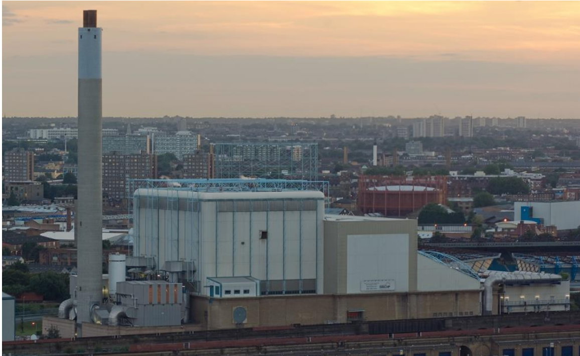
Figure 19: The SELCHP facility
